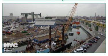
For the last few weeks, DEP has been dredging portions of Newtown Creek. This work, in combination with the arrival of the department's newest sludge boat, which runs shallower than the older models, will allow the boats to navigate the Creek and dock alongside the Newtown Creek Wastewater Treatment Plant in Whale Creek. Once the dredging is completed and the dock is fully constructed, DEP will tear down the existing sludge tank on the Greenpoint waterfront where the sludge boats currently dock.
