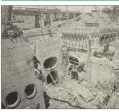
Photo from June 18, 1912 showing the lower gate chamber of the Catskill Aqueduct Headworks, which were a labyrinth of subsurface tunnels and chambers equipped with valves, sluice gates, and operating equipment. They release water from the Ashokan Reservoir into the Catskill Aqueduct and can route millions of gallons of water each day. The lower gate chamber is on the downstream side of the
