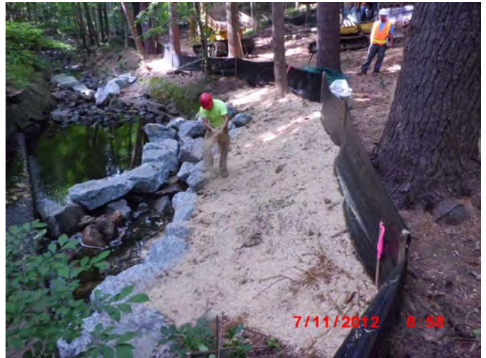
Figure 4.30 Seeding and mulching at Whippoorwill.
