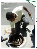
Sheldon exited the facility to inspect the on-site fueling station located in front of the facility. He checked the fill ports for debris and for the required color coding and labels.
