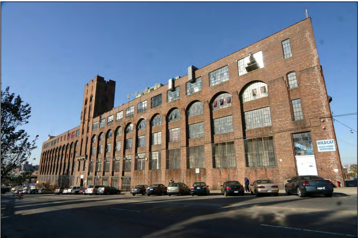
American Bank Note Company Printing Plant (Figure 4): Lafayette Avenue wing, south facade (Photo: Carl Forster)
