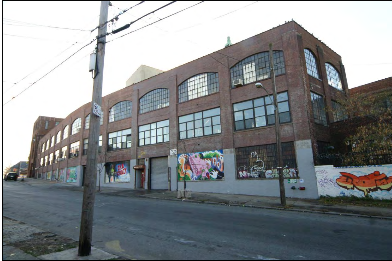
American Bank Note Company Printing Plant (Figure 22): Barretto Street wing, east facade (Photo: Carl Forster)
