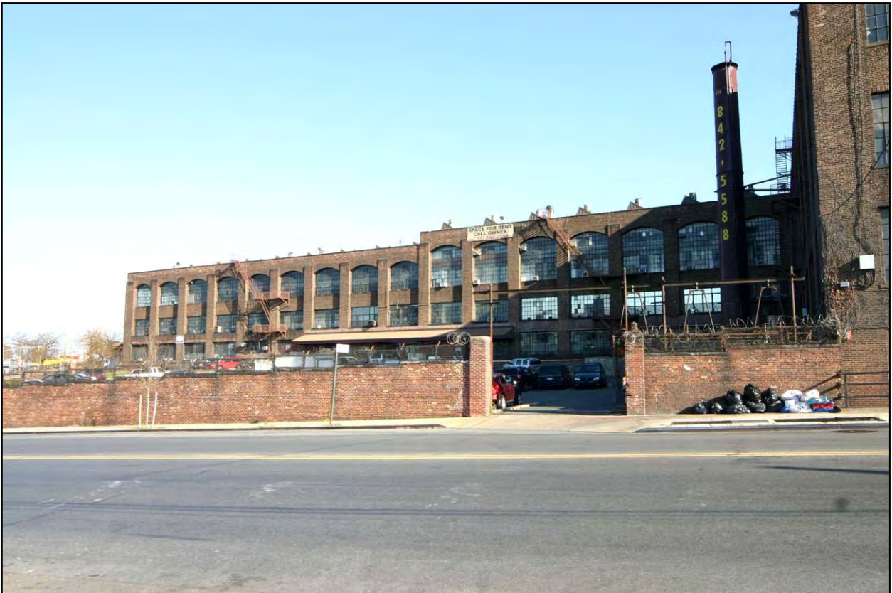
American Bank Note Company Printing Plant (Figure 11): Printing Press wing, west facade, and brick wall (Photo: Carl Forster)
