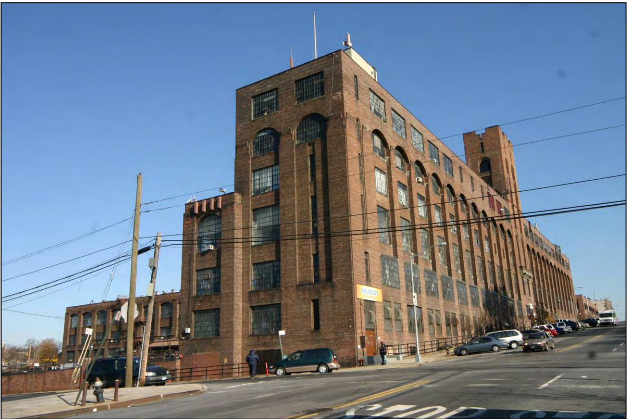
American Bank Note Company Printing Plant (Figure 3): Lafayette Avenue wing, west and south facades (Photo: Carl Forster)
