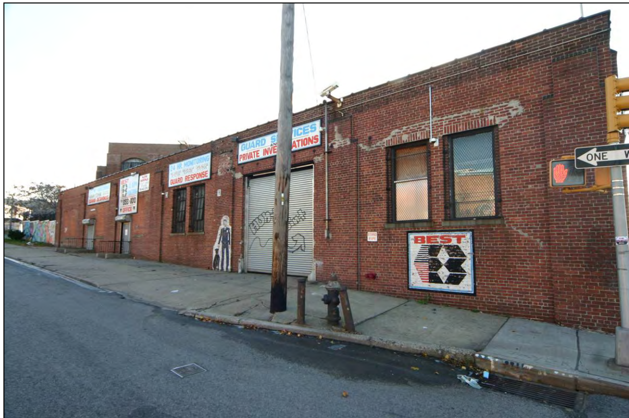
American Bank Note Company Printing Plant (Figure 20): Garage, east facade (Photo: Carl Forster)
