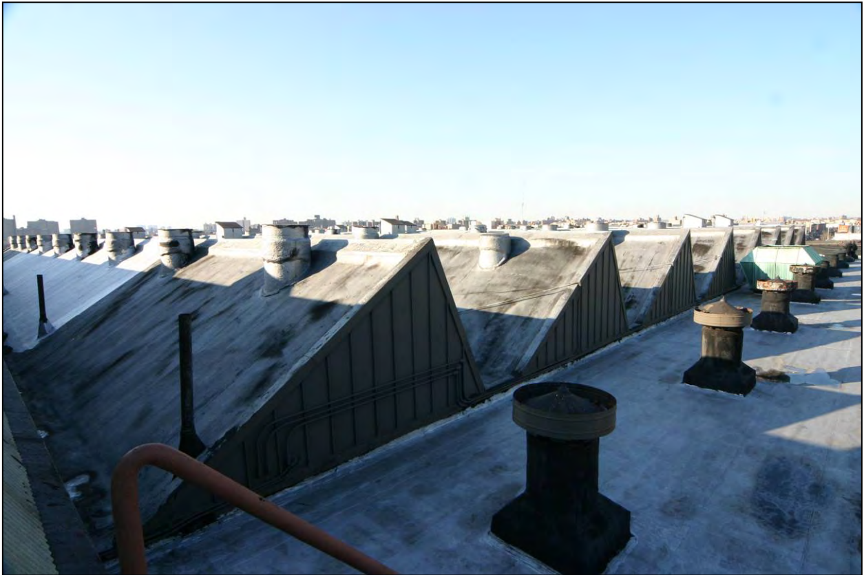
American Bank Note Company Printing Plant (Figure 26): Saw-tooth roof of Printing Press wing (Photo: Carl Forster)
