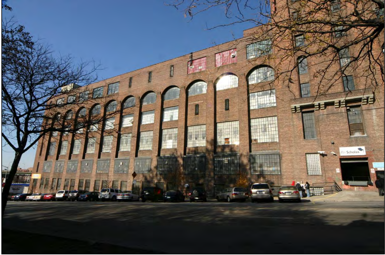
American Bank Note Company Printing Plant (Figure 6): Lafayette Avenue wing, south facade (Photo: Carl Forster)
