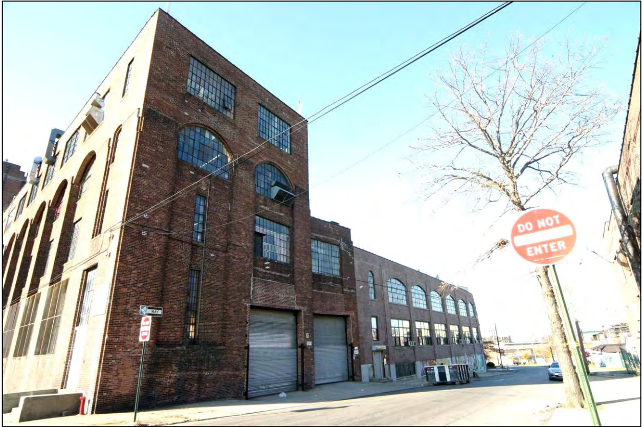
American Bank Note Company Printing Plant (Figure 5): Lafayette Avenue and Barretto Street wings, east facades (Photo: Carl Forster)
