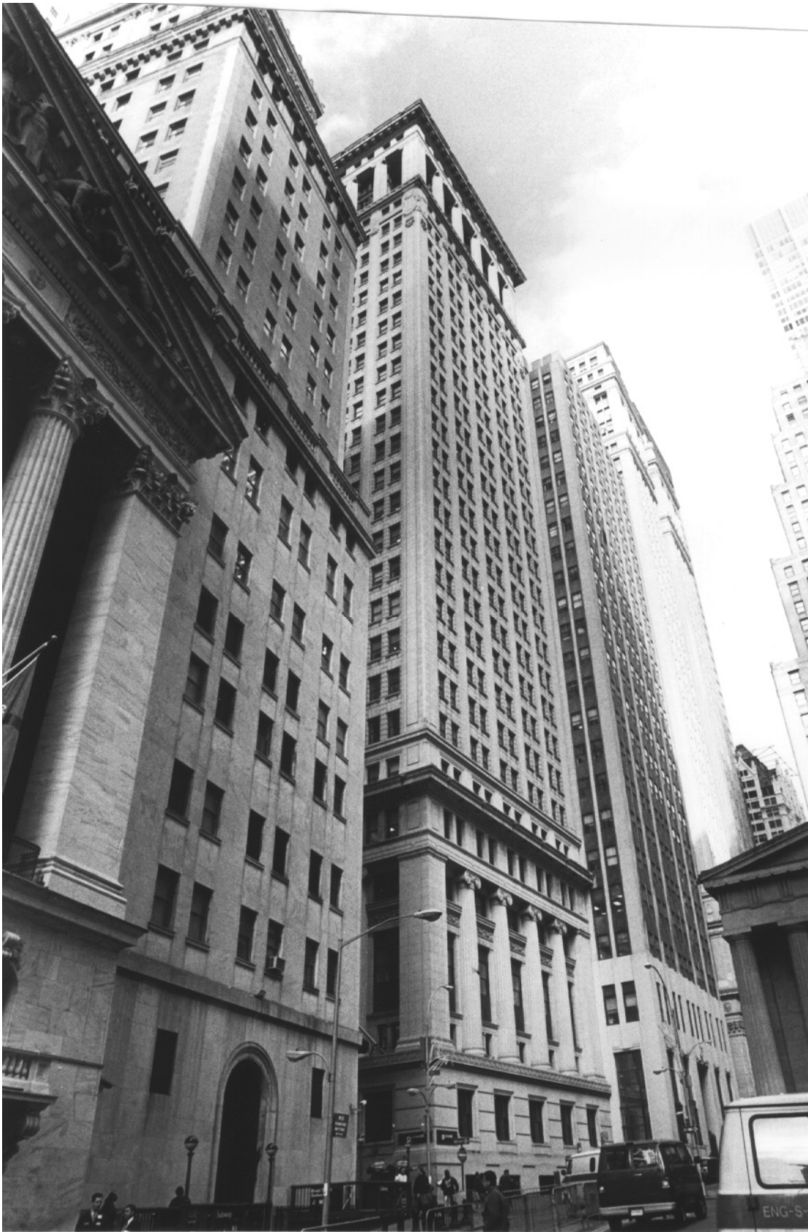
14 Wall Street Building (formerly Bankers Trust Building), 14 Wall Street, Manhattan View from the southeast show the Nassau Street façade
