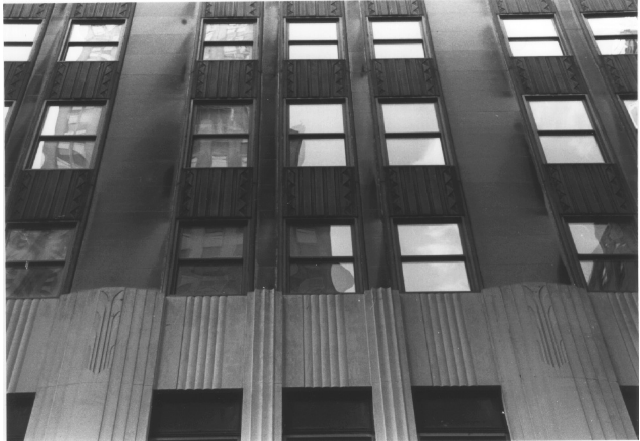
Details of the upper story articulation of the tower (top) and 1930s addition (bottom) on Nassau Street
