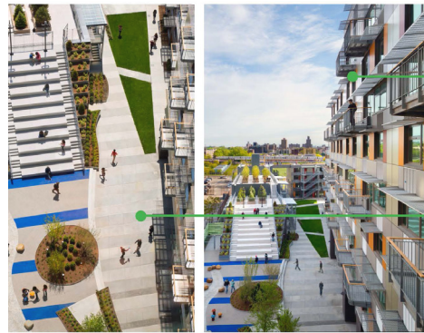
balconies provide per-unit open space that is well integrated into overall building design
