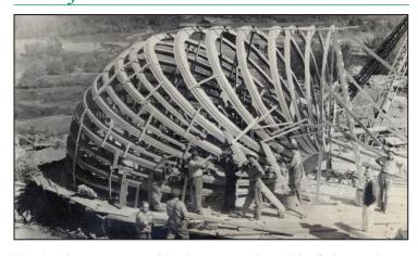
Wooden forms were used in the construction of the Delaware Aqueduct to shape the concrete lining of the tunnel as it was poured. This wooden form was used to mold the gooseneck shape that connected the Rondout Reservoir effluent chamber (where water leaves the reservoir), to the connecting tunnel which led to the first shaft of the Delaware Aqueduct. September 1941.
