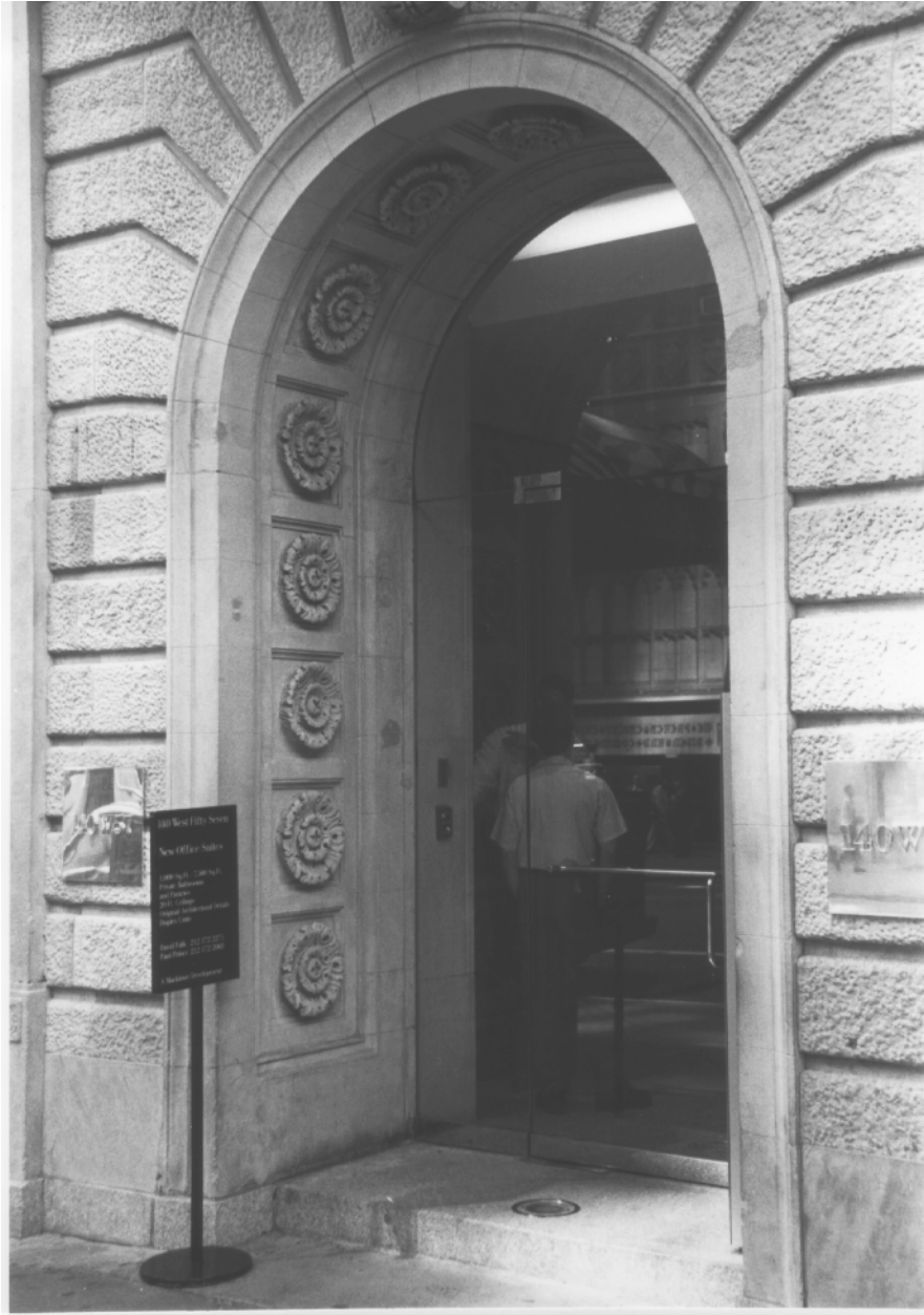
No. 140 West 57 th Street Studio Building Entrance details Photo: Carl Forster
