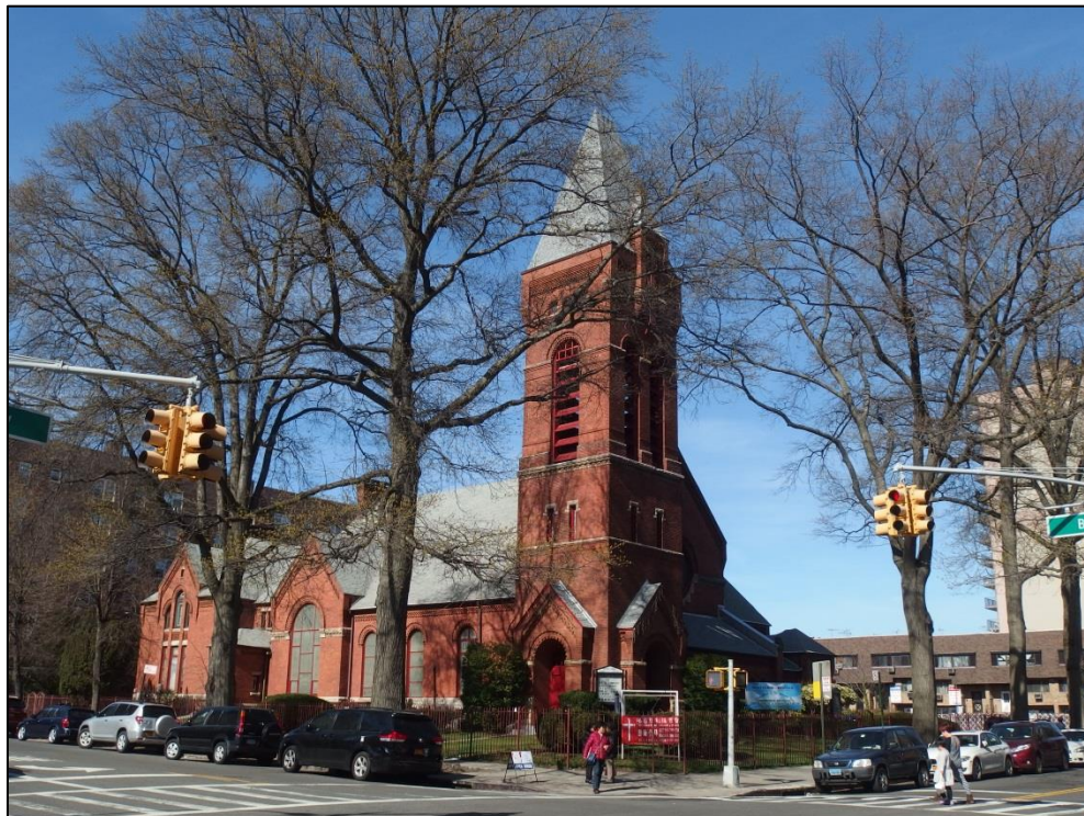
Roosevelt Avenue (South) and Bowne Street (West) Facades (Photograph: Marianne Hurley 2016)
