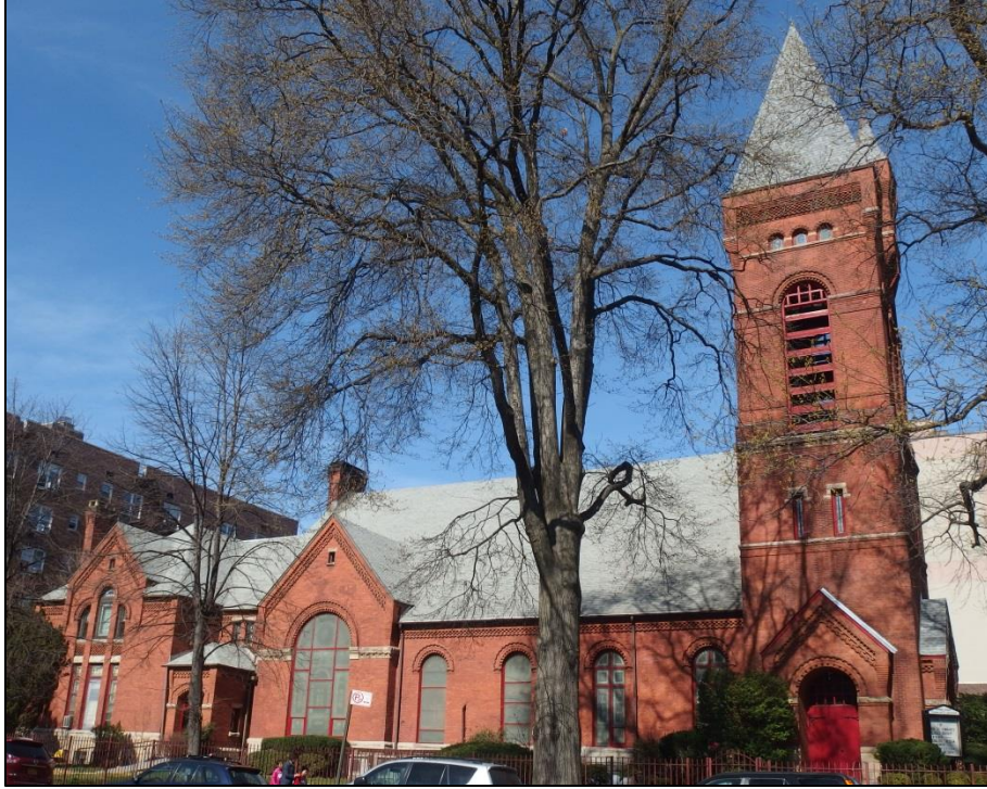
Protestant Reformed Dutch Church of Flushing (Bowne Street Community Church) Bowne Street (West) Facade (Photograph: Marianne Hurley, 2016)
