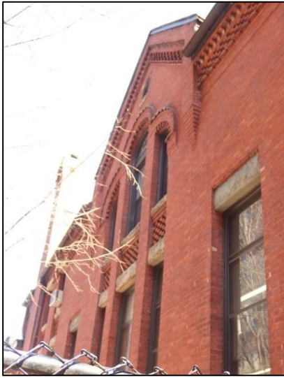
North Facade (details) Transept-like bay at north end (Photograph: Marianne Hurley, 2016)
