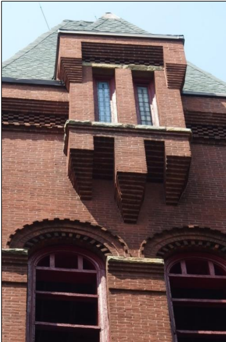
Roosevelt Avenue (South) Facade Tower detail at roof (Photograph: Marianne Hurley, 2016)
