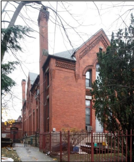
Northwest Corner Transept-like bay at north end (Photograph: Sarah Moses, 2016)
