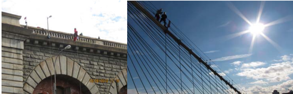
Biennial Inspection in October 2010 – Masonry and Cables.
