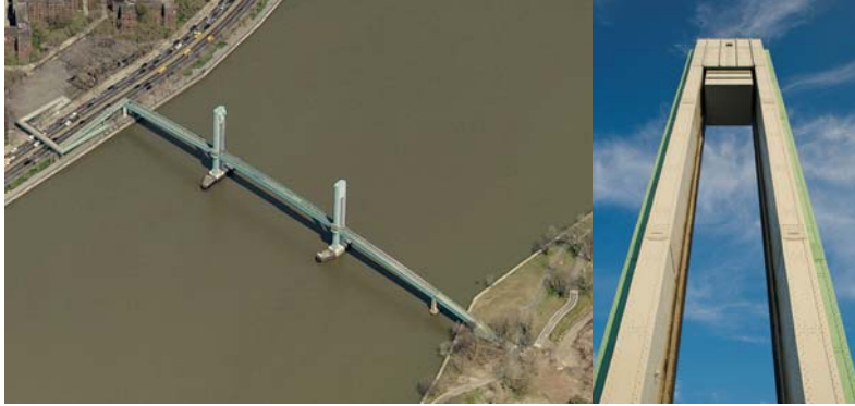
Aerial View. Tower Detail in 2009. (2009 Credit: Duane Bailey-Castro)
