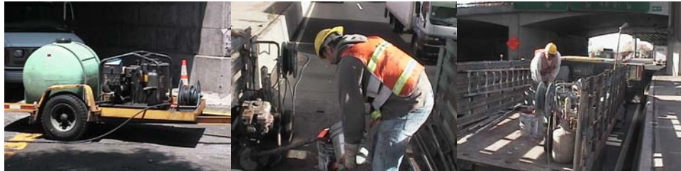
Pressure Washing Machine Used for Graffiti Removal. It is Set to 2500 psi and 212° F. Bridge Painters Frank Duic and Russell Newme Feeding the Spray Pump and Preparing the Paint.
