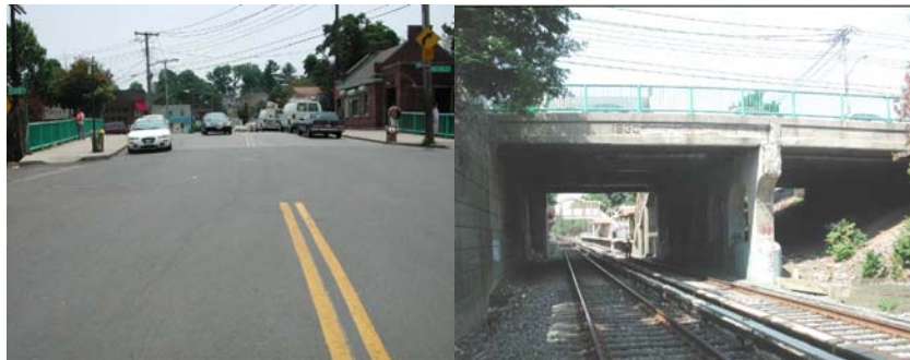
Annadale Road Bridge in 2001. (Credit: NYSDOT)
