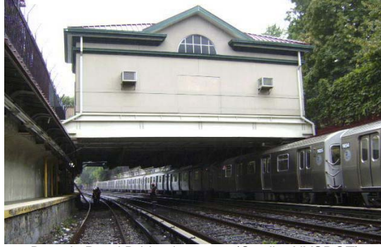
Beverly Road Bridge in 2009. (Credit: NYSDOT)
