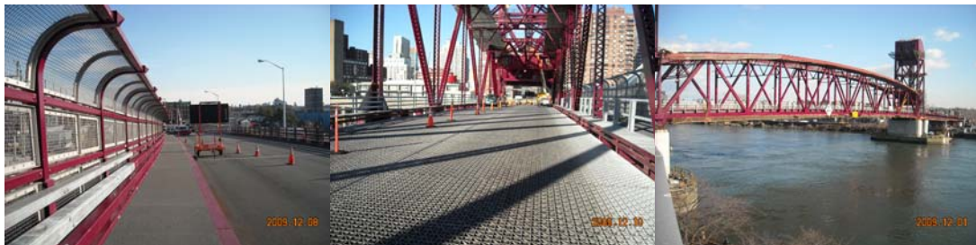
December 2008: East Approach Sidewalk. : Lift Span Open Grid Deck. Lift Span South Elevation
