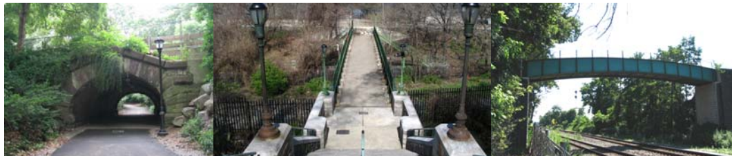
East Drive Bridge over East Wood Arch, West 148 th Street Pedestrian Bridge over Amtrak 30 th Street Branch, Inwood Hill Park Footbridge over Amtrak 30 th Street Branch.
