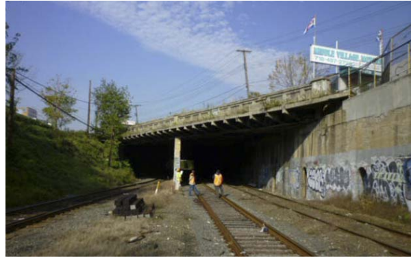
Metropolitan Avenue Bridge in 2009. (Credit: NYSDOT)
