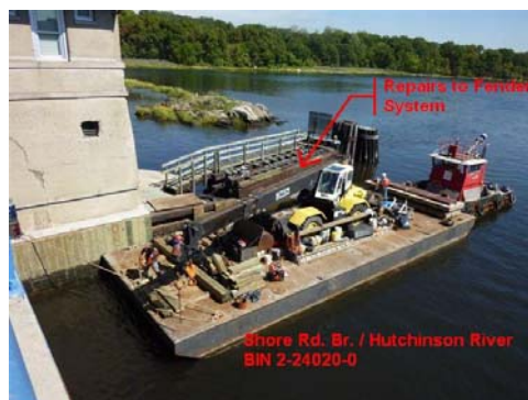
Working on the Shore Road Bridge in September 2010.
