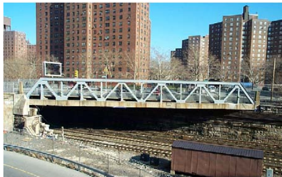
Concourse Village Avenue Bridge. (Credit: NYSDOT)
