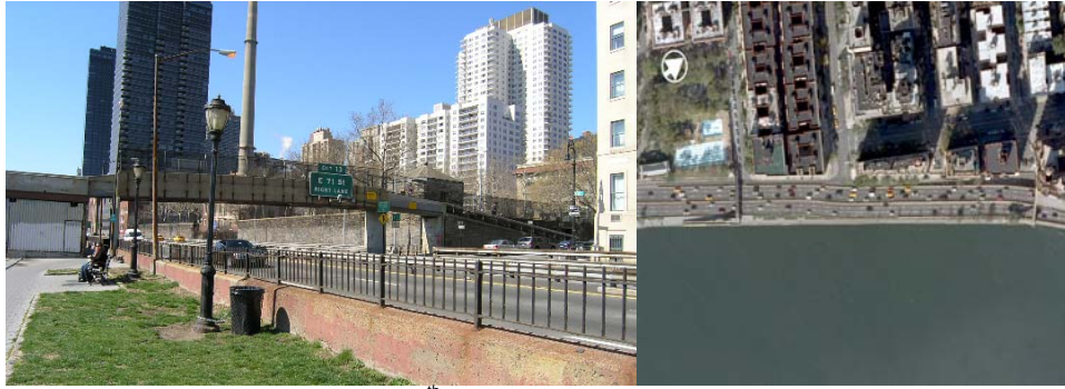
East 78 th Street Bridge. Aerial View.
