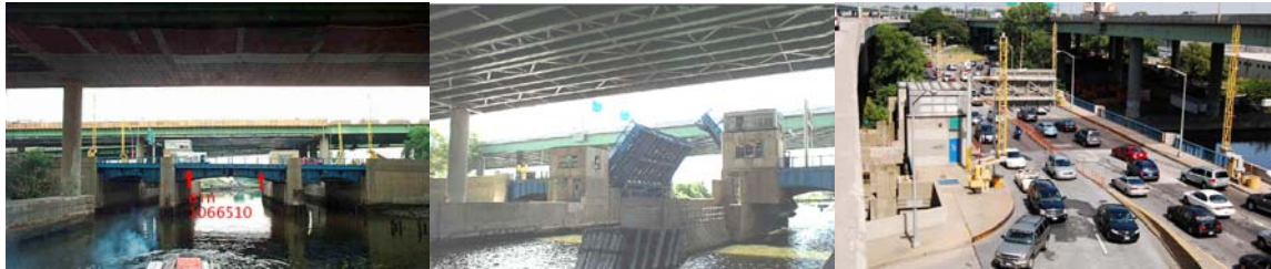
Unionport Bridge in 2002. (Credit: NYSDOT) Eastbound View.
