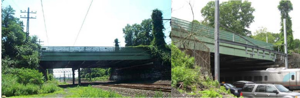
Shore Road Circle Bridge in 2003 and June 2009. (2003 Credit: NYSDOT)
