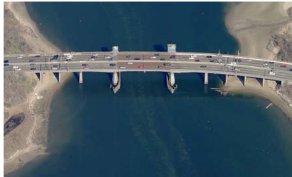
Mill Basin Bridge Aerial View.
