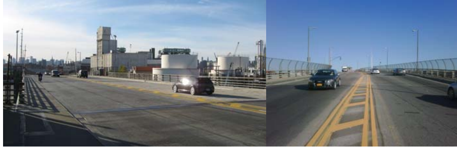
Finished Greenpoint Avenue Bridge Roadway and Sidewalk in November 2010.
