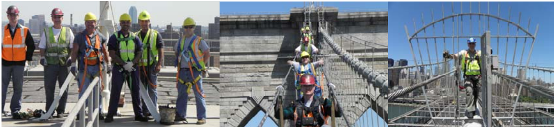
Crew Atop the Brooklyn Bridge in June 2010: Electrician Eugene Kolesnyk, Oilers Stanley Karolewicz, Thomas McAuliffe, Samuel Garcia Jr., and Daniel Cantirino, and Electrician Brian Heaney. (Credit: Thomas Whitehouse) Crew on the Cable. (Credit: Thomas Whitehouse) Executive Director of Bridge Preventive Maintenance and Repair Thomas Whitehouse at the Suicide Gate.
