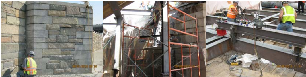
September 2010: Ramp D Demolition and Pre-Stage Work.
