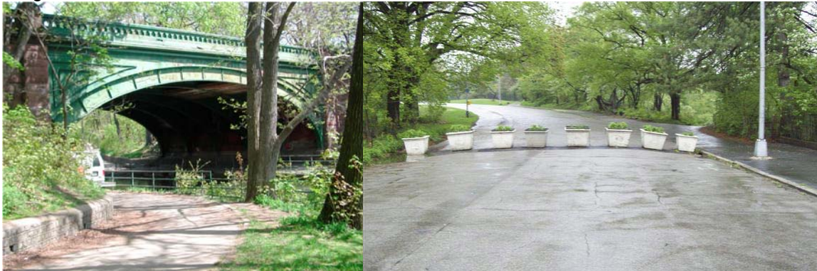
Hill Drive Bridge in 2001. Near End Approach in May 2009: Concrete Flower Pots Close the Roadway. (Credit: NYSDOT)
