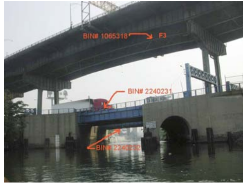
Hamilton Avenue Bridge (#2240231 and 2240232). (Credit: NYSDOT)
