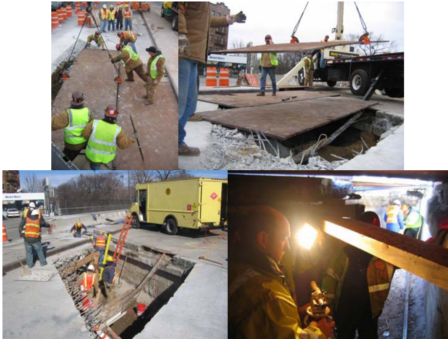
Red Flag Repairs in February 2006: Ironworkers Removed the Plates From the Holes and Replaced Them at the End of Each Day. They Also Placed Reinforcing Bars for the New Concrete Slab. Supervisor Bridge Repairer and Riveter Gean Pilipiak Monitoring Red Flag Repairs in 2006. (Credit: Peter Basich)
