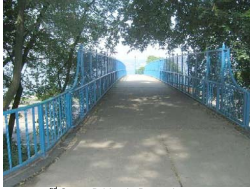
92 nd Street Bridge in December 2006.
