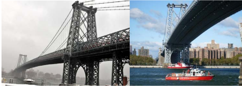
Williamsburg Bridge in February 2010. (Credit: Samuel Teaw). October 2010: FDNY Boats at Bridge Tower Bases During Testing.
