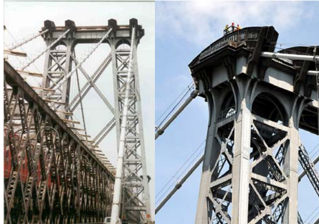
Williamsburg Bridge in 2003. (Credit: Peter Basich) Tower Detail in 2009. (Credit: Bernard Ente)
