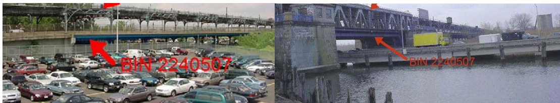
Roosevelt Avenue Bridge (#2240507) in 2002 and 2004. (Credit: NYSDOT)
