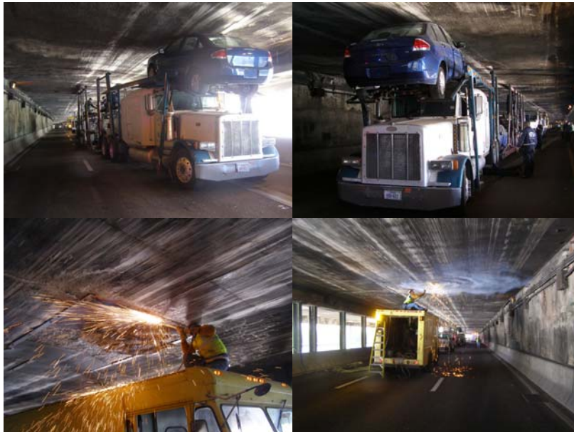
Division Ironworkers Removing Loose Metal Strips Under the Promenade.
