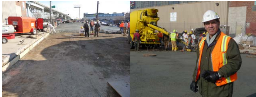
December 2010: Concrete Work. Associate Project Manager Reza Lotfi. (Credit: Leonid Gitis)
