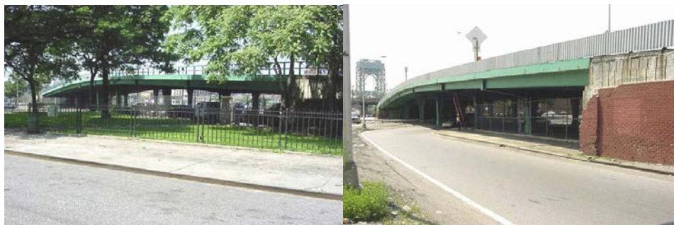
Left and Right Views of the Bridge in 2003.
