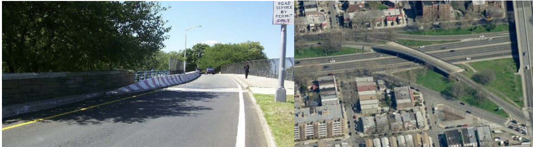
September 2009: Top of Deck Along Left Shoulder. (Credit: NYSDOT) Aerial View in 2009.
