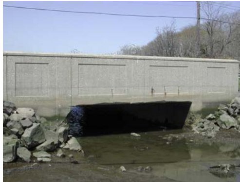
Arthur Kill Road Bridge in 2009. (Credit: NYSDOT)
