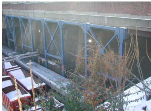
West 31 st Street Bridge in 2004. (Credit: NYSDOT)
