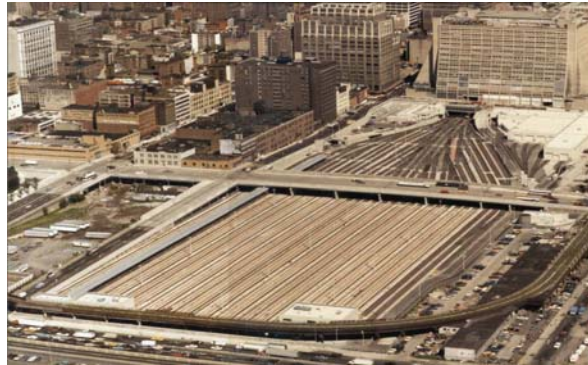
11 th Avenue Viaduct Site Overview.
