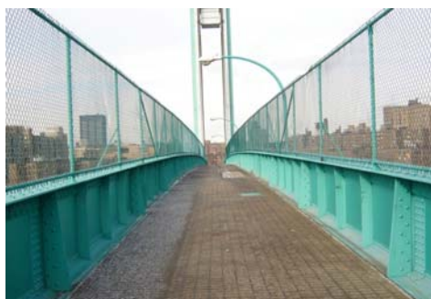
Existing Concrete Deck.
