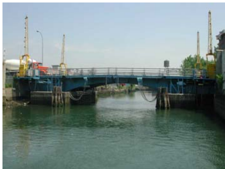
3 rd Street Bridge in 2009. (Credit: NYSDOT)
