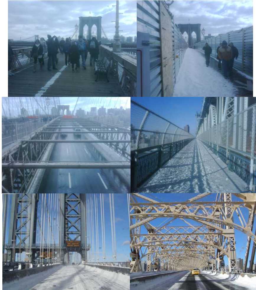
Brooklyn Bridge Cleared After the Blizzard. Manhattan Bridge Walkway. (Credit: Russell Holcomb) Manhattan Bridge and Queensboro Bridge Roadways. (Credit: Bojidar Yanev)
