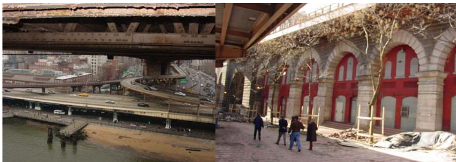
Brooklyn Bridge Ramps and Arches in November 2008. (Credit: Maria Mikolajczyk)
