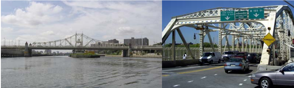
Macombs Dam Bridge (Elevation Credit: NYSDOT).
