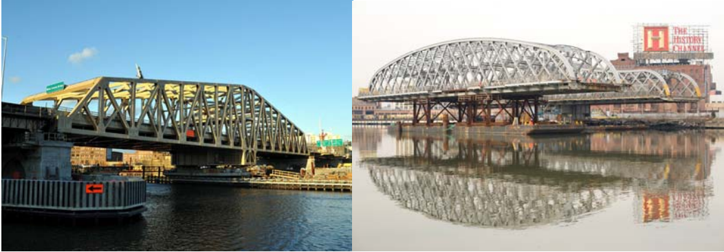
New Span in November 2010. (Credit: Bernard Ente) Old Willis Avenue Spans in December 2010. (Credit: Duane Bailey-Castro)
