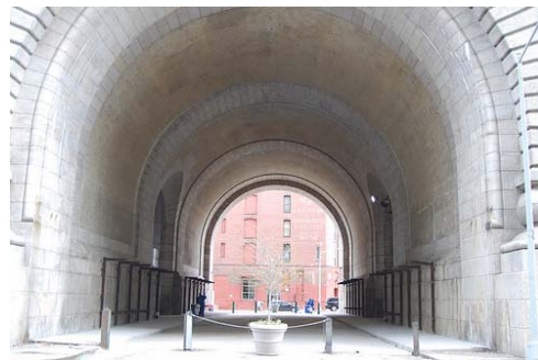
Completely Repaired Water Street Arch in April 2009. (Credit: DUMBO NYC)
