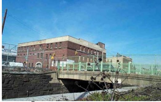
East 175 th Street Bridge in 2002. (Credit: NYSDOT)
