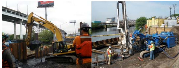
Removal of Obstructions for the Sheeting Operation in May 2009. Deep Well Installation Southwest of the Bridge in June 2009.
