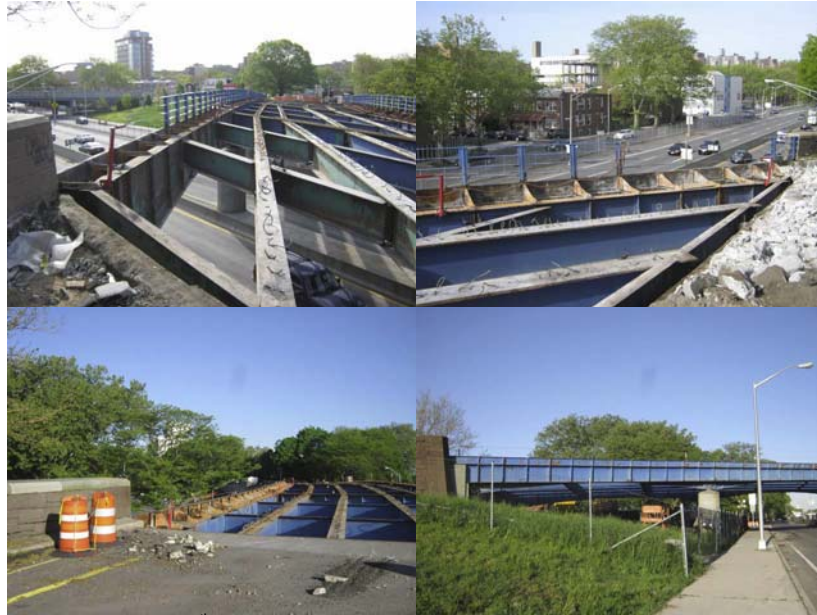
East 8 th Street Bridge Rail Removal in April and May 2010.
