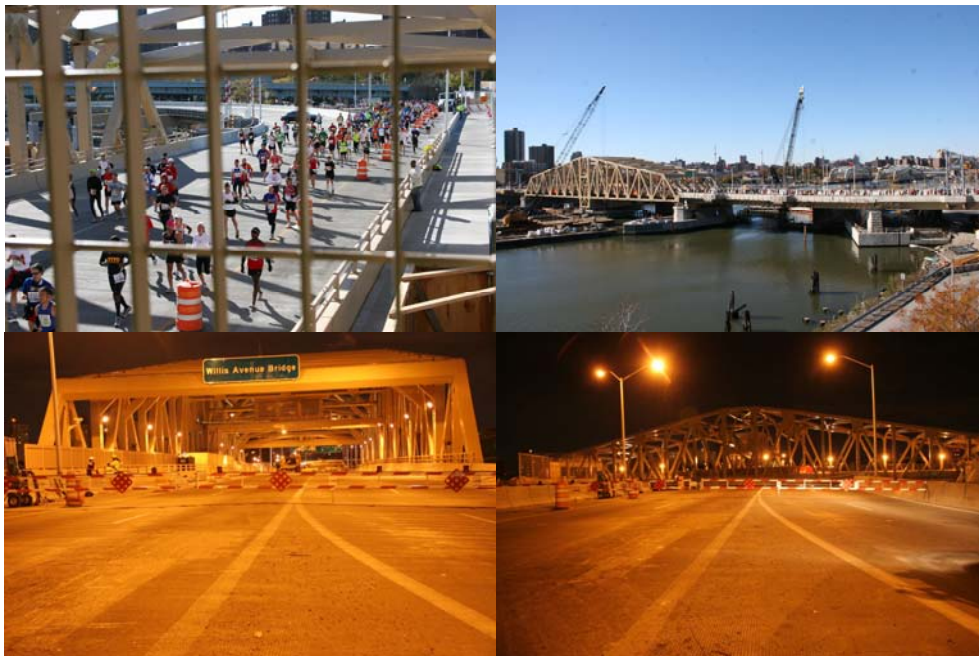
NYC Marathon Runners on the New Bridge in November 2010. First Test Operation of the New Span in December.
