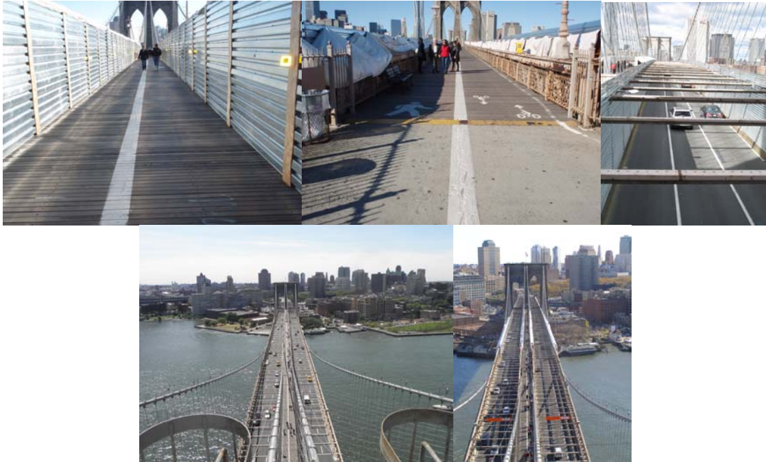
Bicycle/Pedestrian Path with Protective Shielding and Containment in November 2010. Roadway Shielding in October 2010. Main Span View in June and November 2010. (June Span Credit: Thomas Whitehouse. November Span Credit: Bojidar Yanev)
