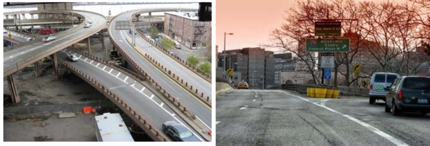
Ramps A , C, and F Will be Widened.
