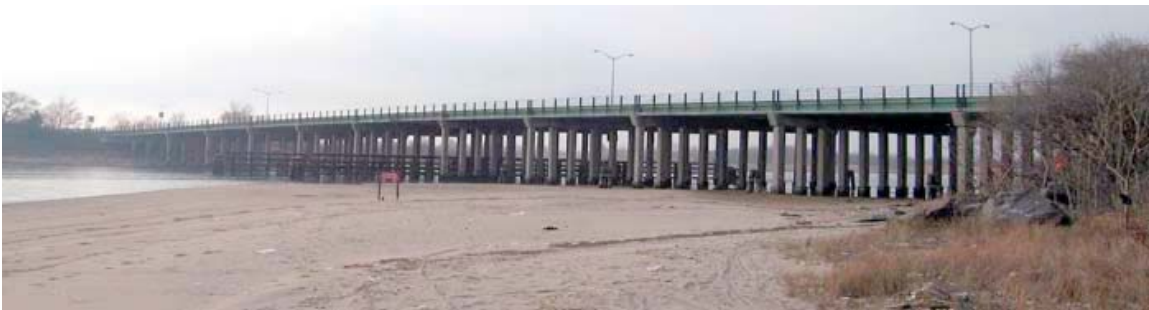
Paerdegat Basin Bridge.
