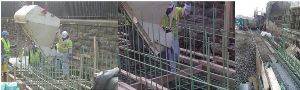
Concrete Placement in Late 2010.
