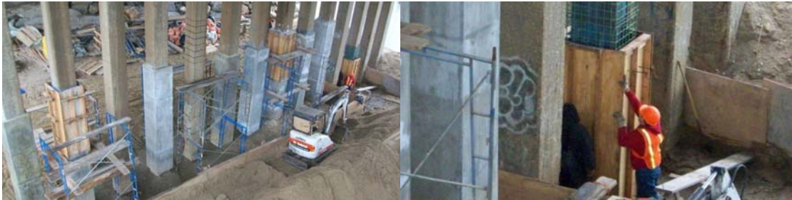
Pier 3 Column Repair in December 2008. (Credit: NYSDOT)
