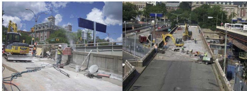
June 2010: Ramp A and D Demolition.
