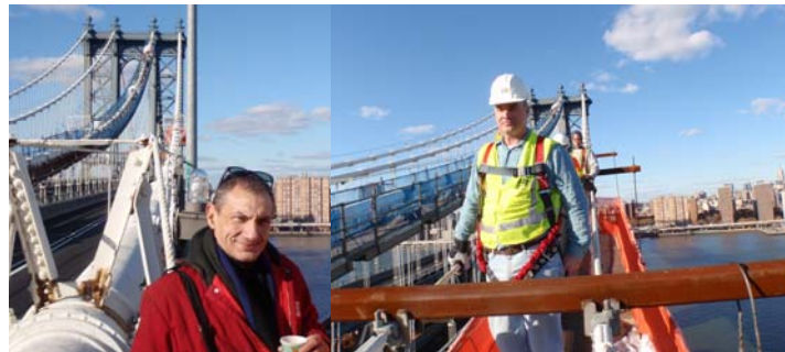
Executive Director of Bridge Inspections and Bridge Management Dr. Bojidar Yanev. (Yanev Credit: Brian Gill) Manhattan Bridge Engineer-in-Charge Brian Gill Inspecting Cable "D."
