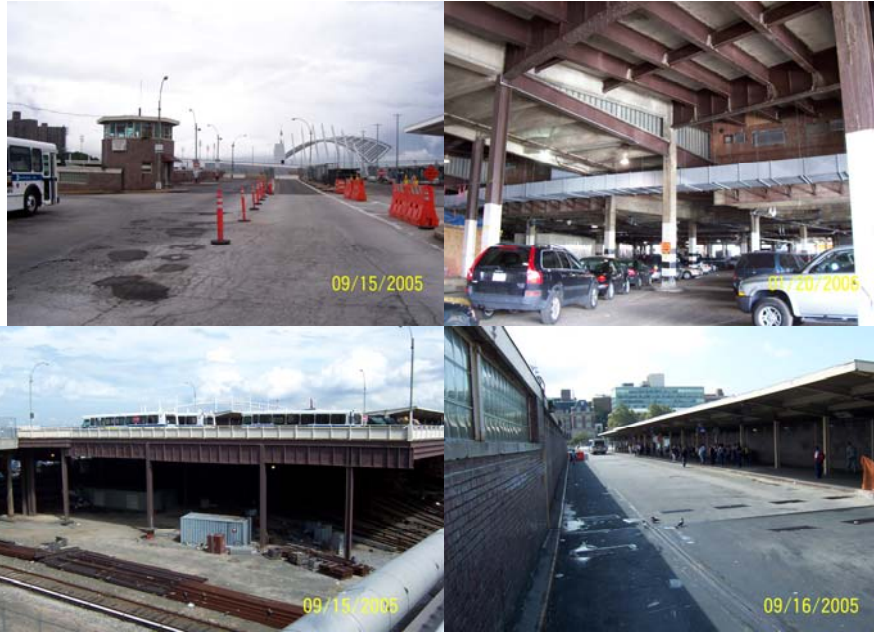
Bus Station North - over Terminal Building, SIRT Station and Employee Parking Lot. Station South - over SIRT Station and Employee Parking Lot.
