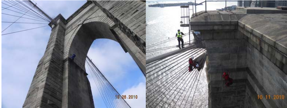
Brooklyn Bridge Biennial Inspection in October 2010.
