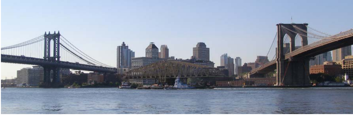
Voyage up the East River on July 26, 2010. New Willis Avenue Bridge Span Between the Manhattan and Brooklyn Bridges. (Credit: Bojidar Yanev)
