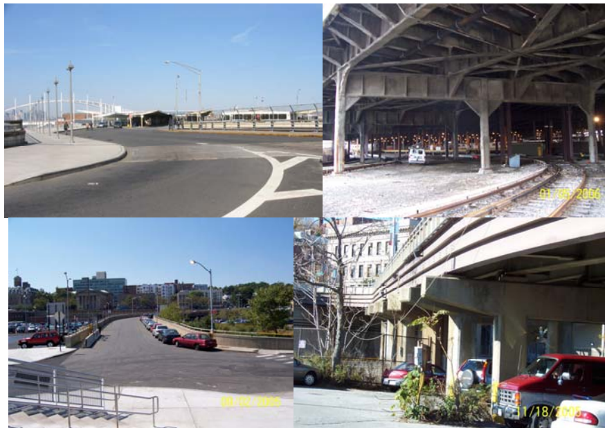
Old Viaduct - Bus Exit over SIRT Tracks. North Ramp - over SIRT Tracks and North Municipal Parking Field.
