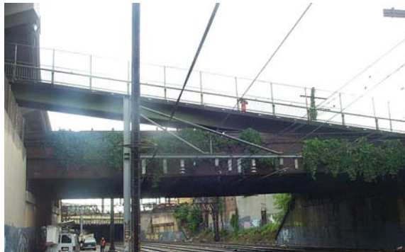
Bryant Avenue Bridge in 2002. (Credit: NYSDOT)
