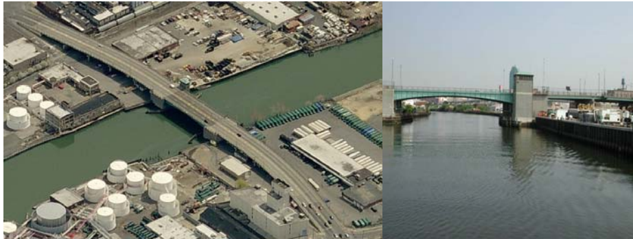
Arial View of Greenpoint Avenue Bridge. Elevation Right Span.
