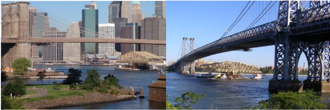
New Willis Avenue Span Passing Under the Brooklyn Bridge. Passing Under the Williamsburg Bridge. (Williamsburg Credit: Ronald Rauch)
