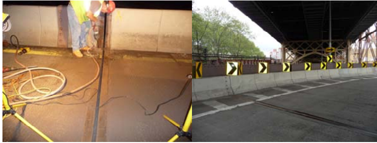
Working on Ramp F in August 2009. Completed Ramp in April 2010.
