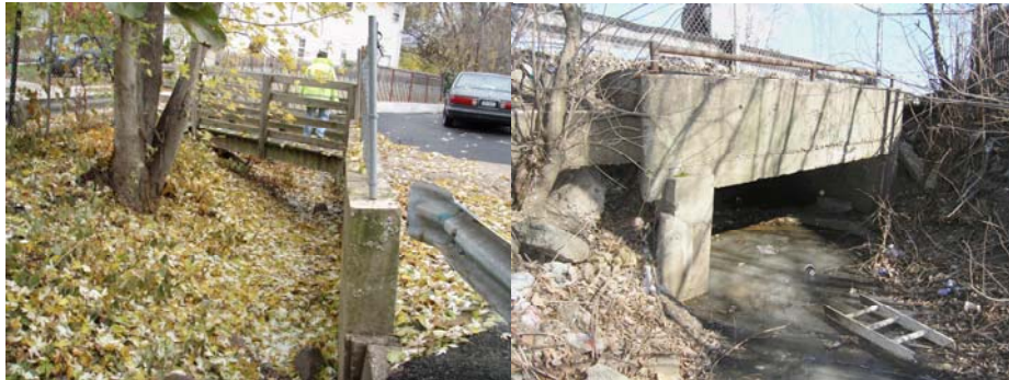
Galloway Avenue over Marianne Street, Forest Avenue over Crystal Avenue.
