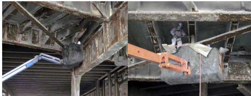
April 2010: Removal of Concrete Encasement Packets at the Old Viaduct.
