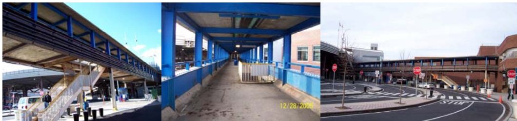
Pedestrian Breezeway - Over Commuter Drop-Off / Pick-Up Area.
