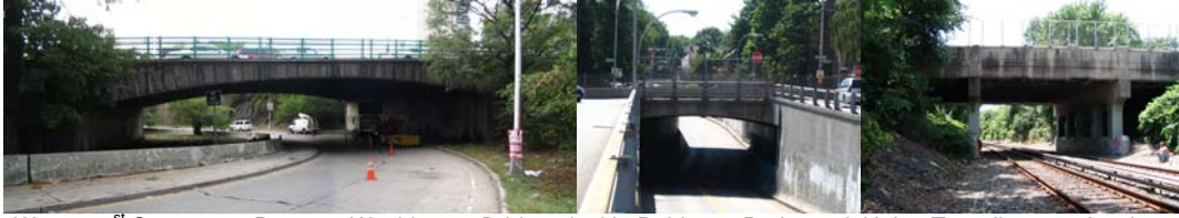
West 181 st Street over Ramp to Washington Bridge, Jackie Robinson Parkway & Union Turnpike over Austin Street, Albee Avenue Bridge over SIRT South Shore.
