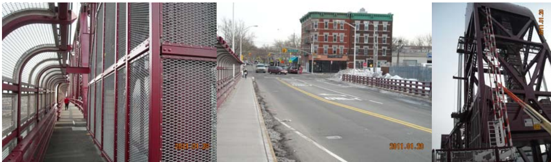
Roosevelt Island: North Sidewalk With New Pedestrian Fence. Vernon Boulevard and 36 th Avenue Intersection With New Turn Lane. Recently Painted Bridge With New Traffic Control Equipment.
