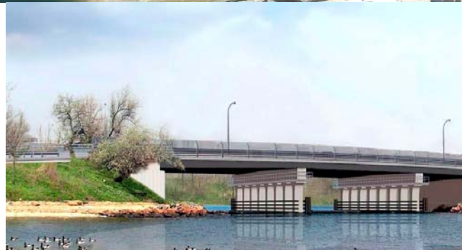
Fresh Creek Bridge Aerial View and in 2002. (2002 Credit: NYSDOT) Proposed Fresh Creek Bridge.
