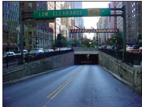
Park Avenue Tunnel in 2003. (Credit: NYSDOT)
