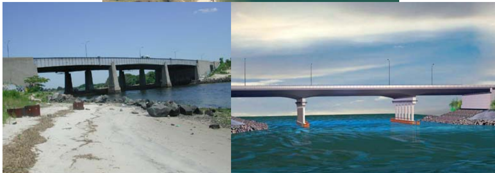
Gerritsen Inlet Bridge Aerial View and in 2002. (2002 Credit: NYSDOT) Proposed Gerritsen Inlet Bridge.
