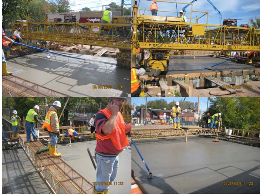
Annadale Road Bridge: Placing the Concrete Deck in October 2009.
