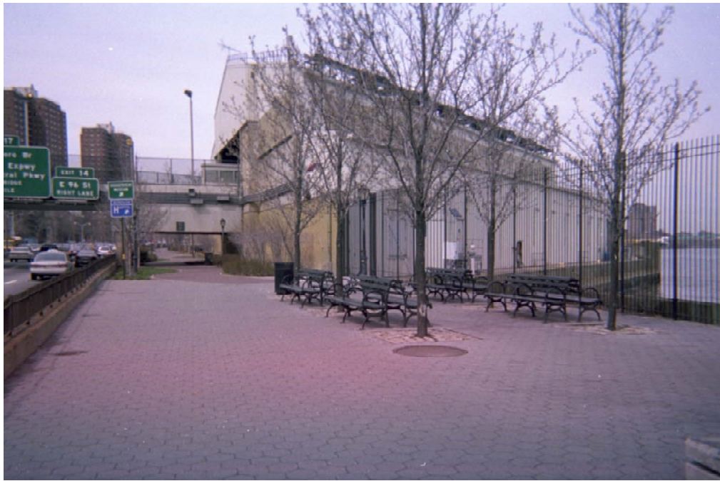
Figure 10.7-1 : View of East 91st Street MTS from adjacent East River Esplanade.
