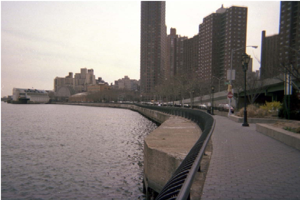
Figure 10.7-6 : View south toward East 91st Street MTS from East River Esplanade at East 96th Street.
