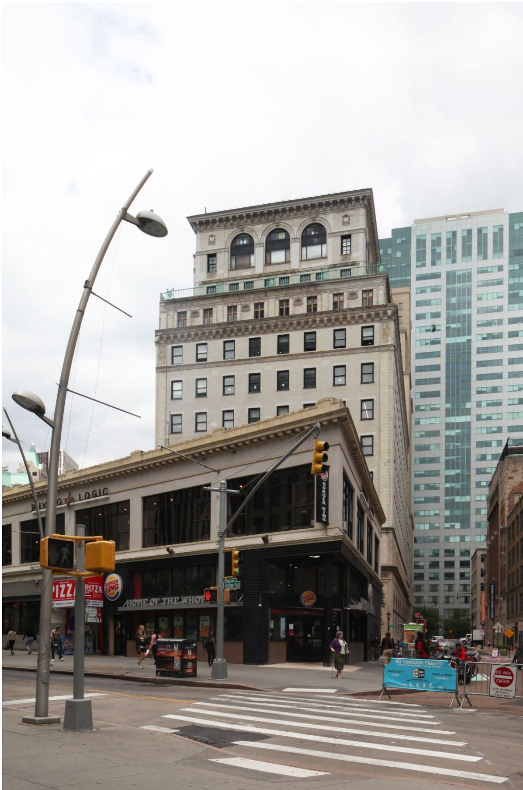
South facade of the Brooklyn Edison Building, from the intersection of Fulton and Pearl Streets
