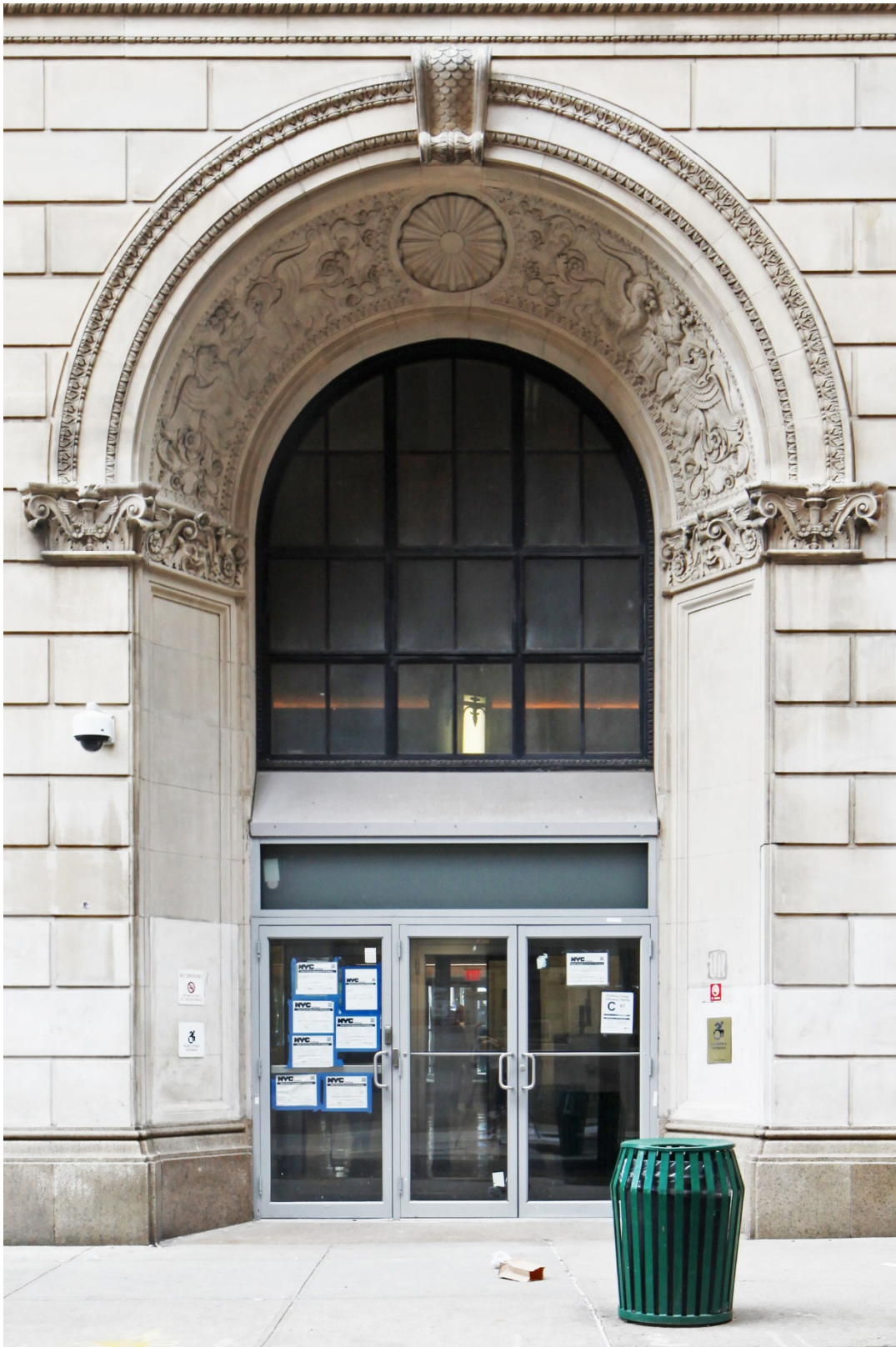
Main entrance on Pearl Street with highly elaborate Renaissance Revival style intrado
