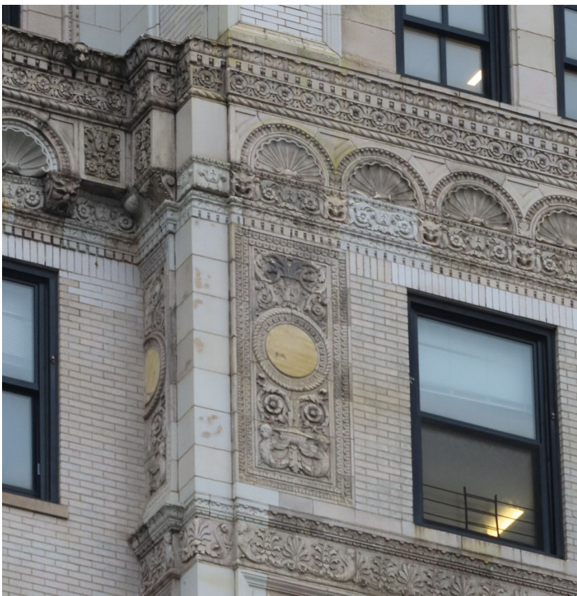
Renaissance Revival style terra-cotta details on the ninth story of the Adams Street facade
