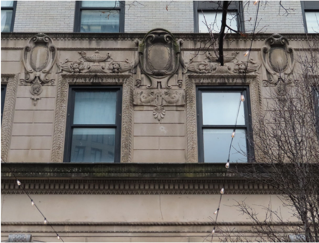
Renaissance Revival style cartouches and festoons on the Pearl Street facade
