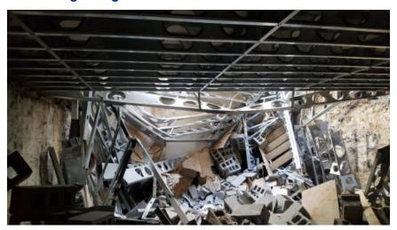
Following the tragic worker fatality earlier this year due to a building collapse caused by overloading of cold-formed steel, the Department is reminding contractors that overloading and improper installation of cold-formed steel including joists, rafters, trusses, and structural wall studs, etc., can result in injury and property damage.
