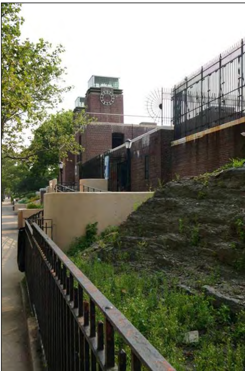
Crotona Play Center: Fulton Avenue (view north) (l); Fulton Avenue Ancillary Stairs (r), Borough of the Bronx
