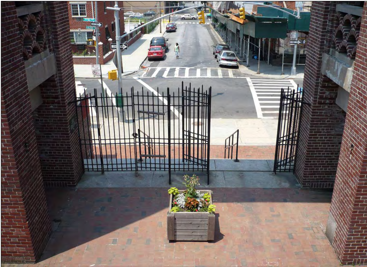
Crotona Play Center: Entrance Courtyard, Main Gates (view west), Borough of the Bronx
