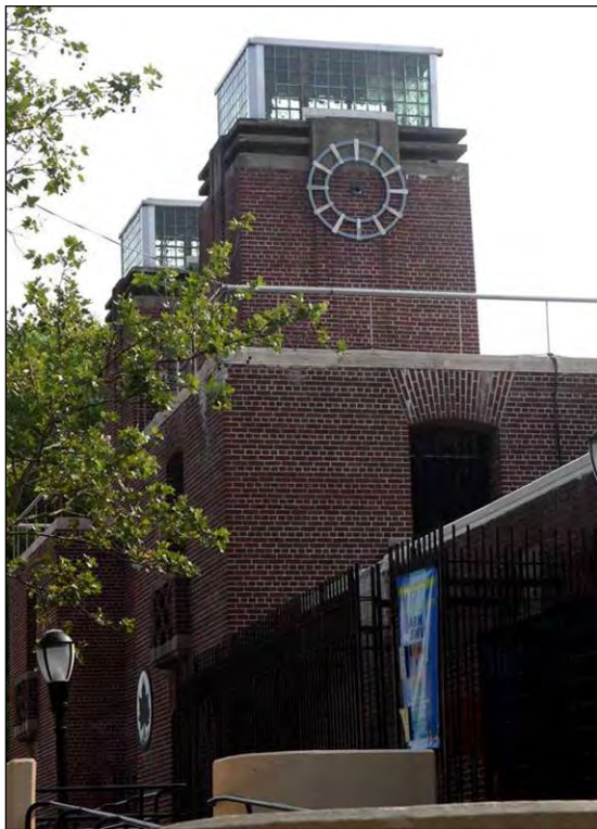
Crotona Play Center: Main Entrance, Fulton Avenue (view northeast) (l); Main Entrance Archway Openings from Second Story (view north) (r), Borough of the Bronx
