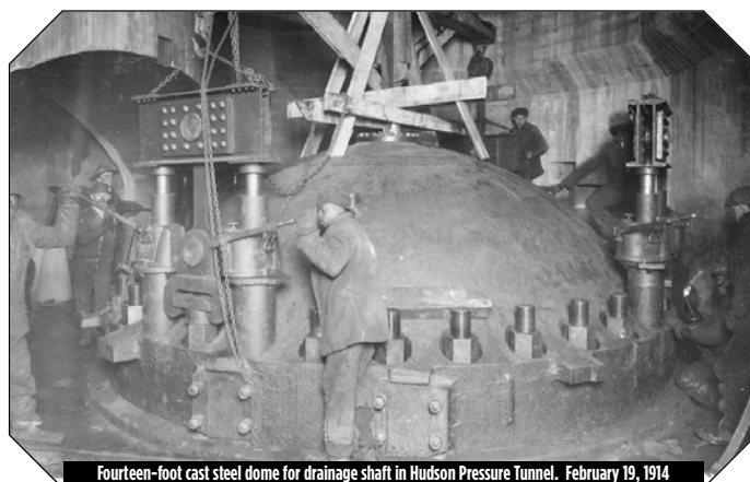
Fourteen-foot cast steel dome for drainage shaft in Hudson Pressure Tunnel. February 19, 1914
