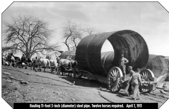
Hauling 11-foot 3-inch (diameter) steel pipe. Twelve horses required. April 7, 1911
