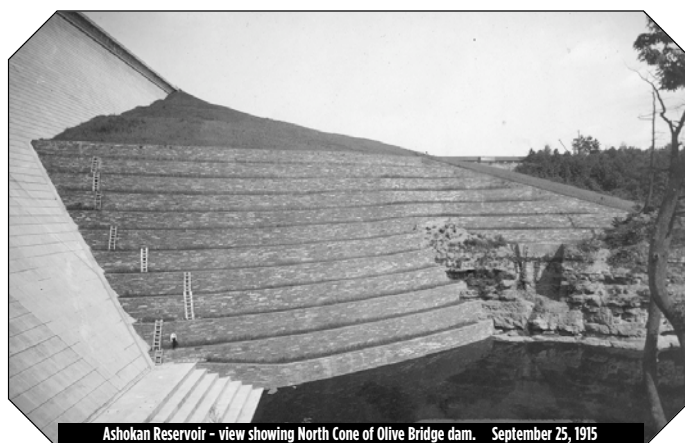
Ashokan Reservoir - view showing North Cone of Olive Bridge dam. September 25, 1915
