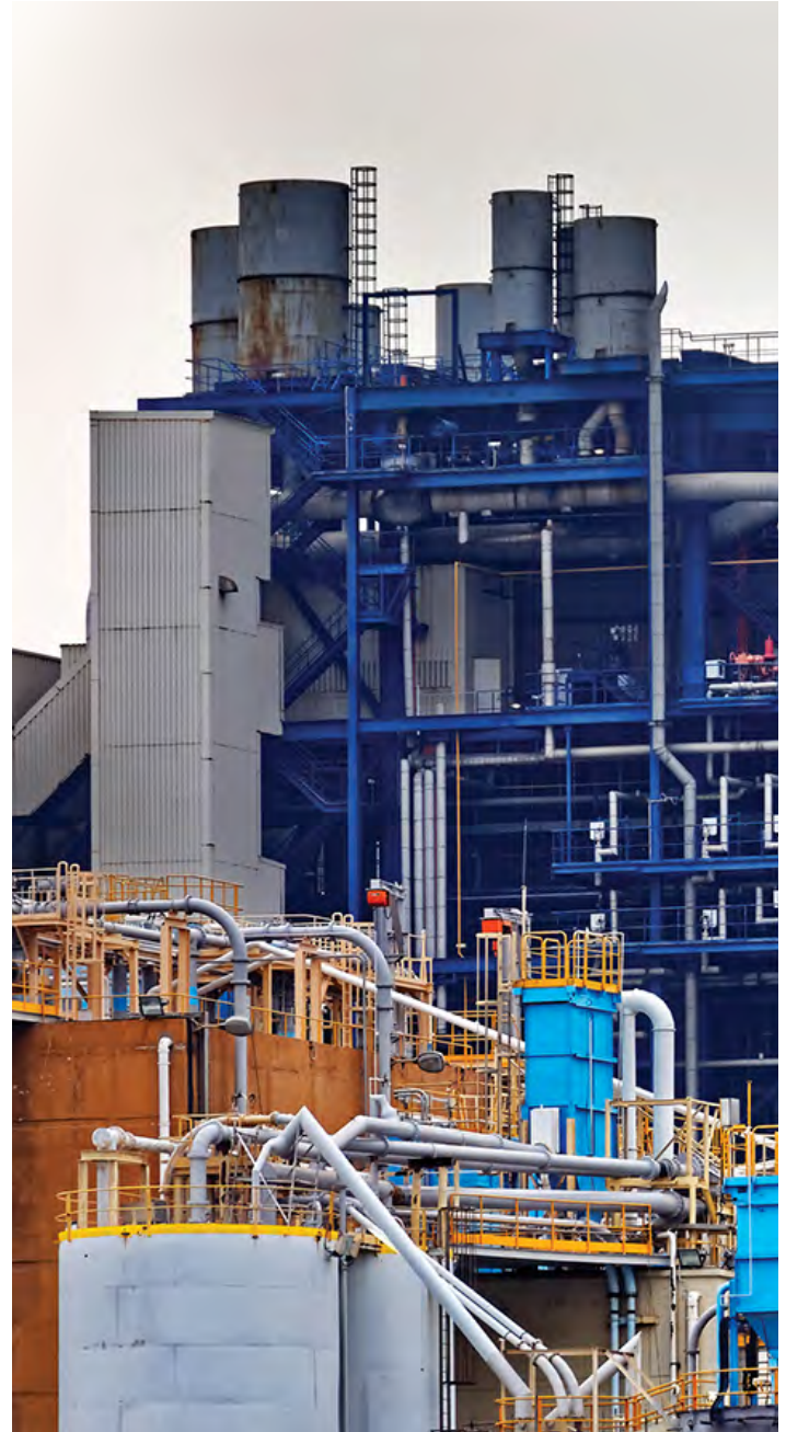
Example industrial facility
