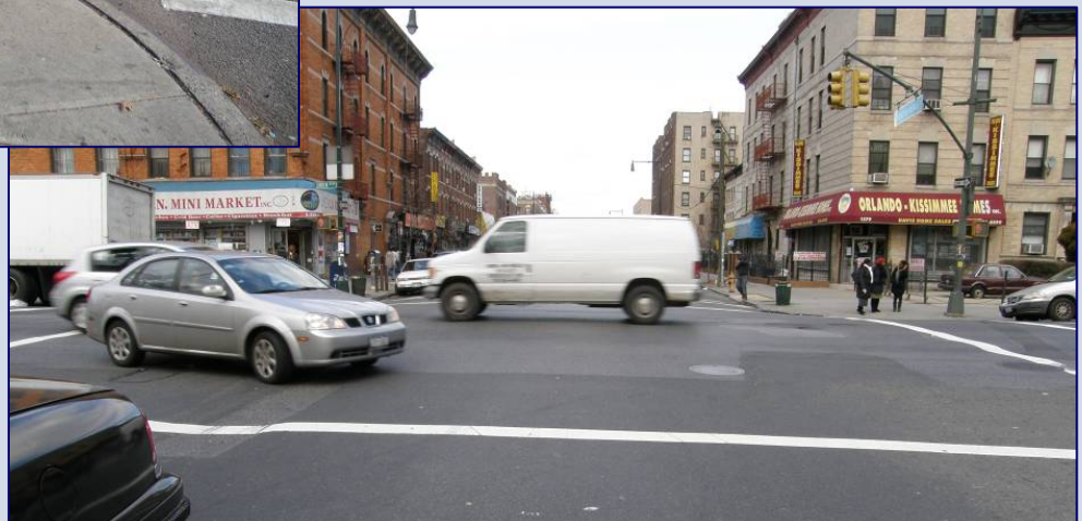
Linden Boulevard and Nostrand Avenue facing north – peg-a-trac will help guide turning movements
