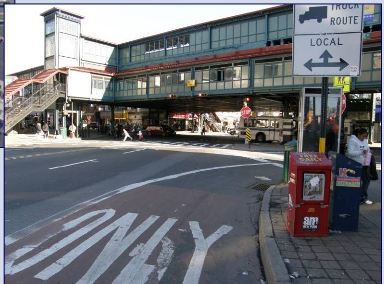
East Fordham Road free right turn onto Jerome Avenue with uncontrolled crossing
