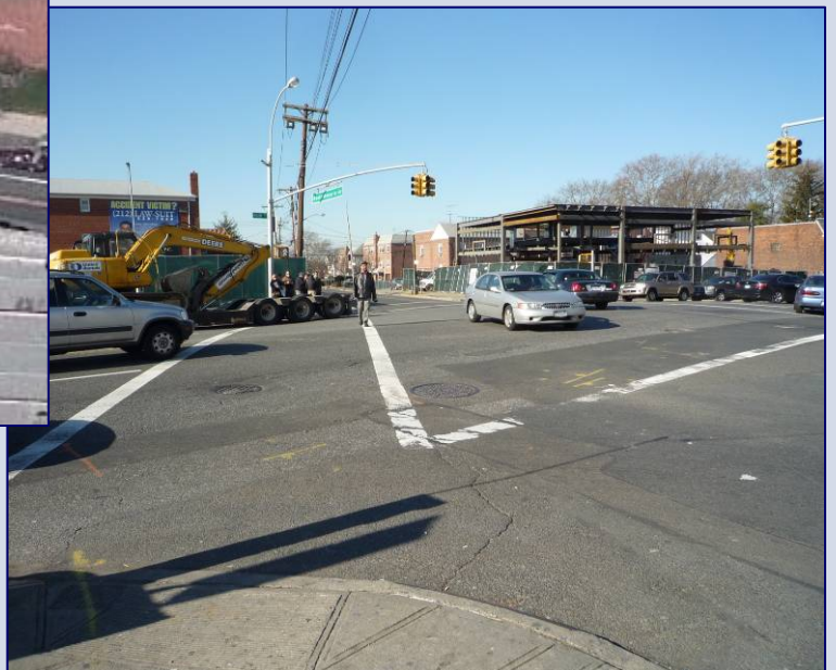
Booth Memorial Avenue at Main Street facing west – Skewed crosswalks create long crossing distances
