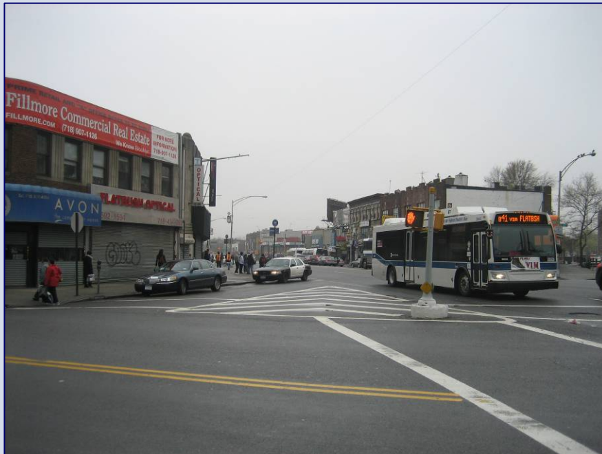
Flatbush Avenue and Avenue H facing north – current painted slip configuration provides no protection to pedestrians waiting to cross Flatbush Avenue
