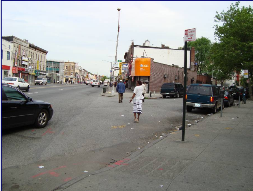
Flatbush Avenue and East 31 st Street facing north – construction of a neckdown and installation of crosswalk will provide more protection for pedestrians from turning vehicles
