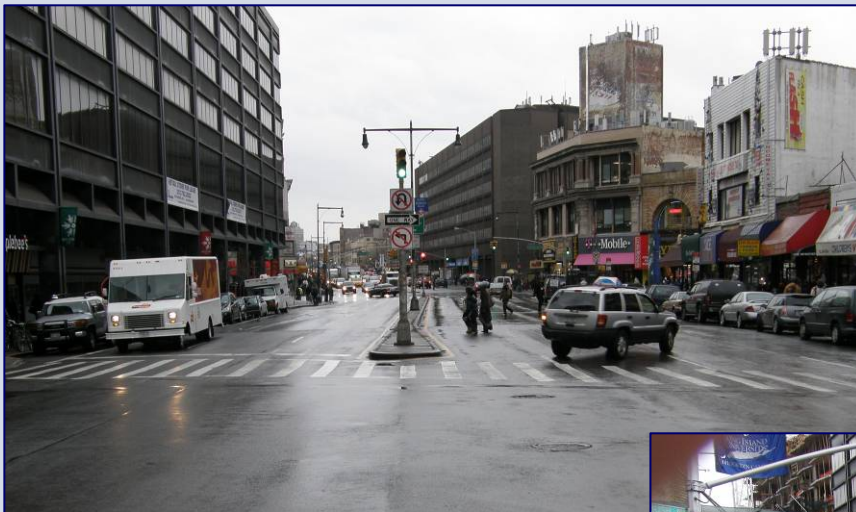
Flatbush Avenue Extension at DeKalb Avenue facing south – a median tip will be extended through the crosswalk to provide more pedestrian protection
