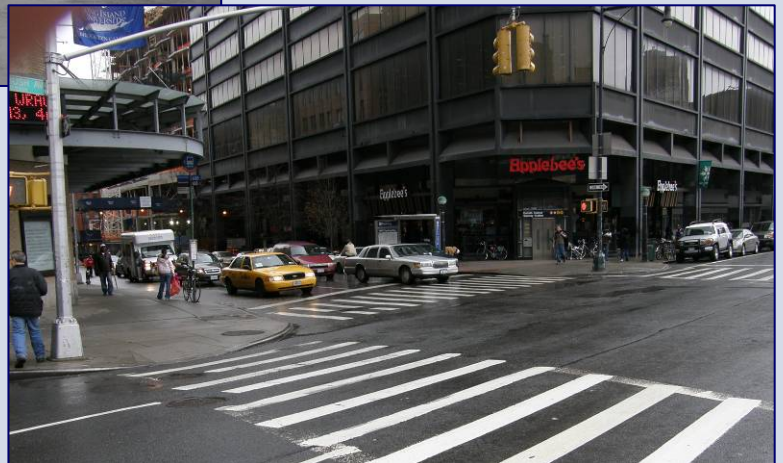
DeKalb Avenue and Flatbush Avenue Extension facing southeast – DeKalb road width will be reduced and sidewalks widened
