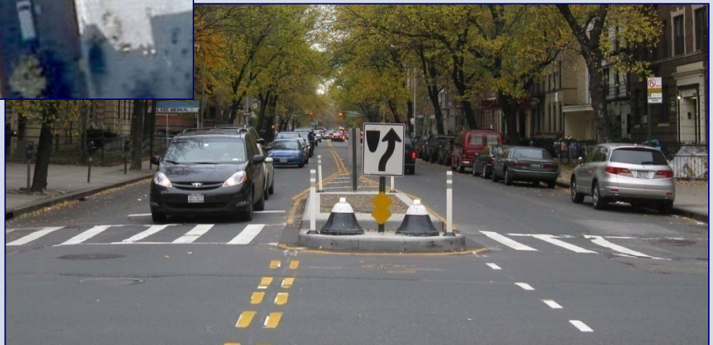
Ocean Avenue Island – This island implemented in 2009 gives pedestrians protection from turning vehicles and a safe place to wait if they are unable to cross the street in one cycle.
