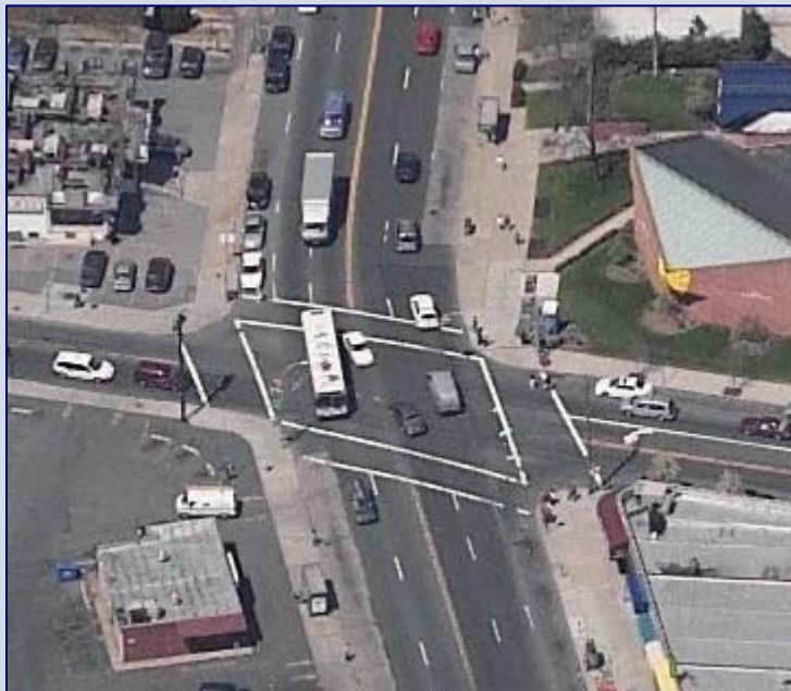
Booth Memorial Avenue and Main Street
