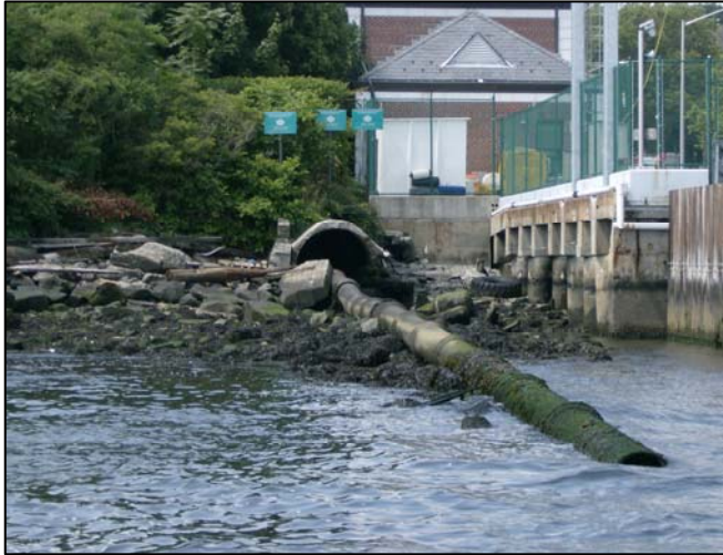
Outfall ID: PR-023A Location: NAUTILUS STREET Latitude: 40° 36' 43" Longitude: 74° 3' 36" Outfall Size: 20" DIA Receiving Water: UPPER NEW YORK BAY
