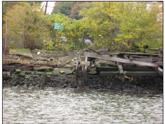
Outfall ID: PR-009 Location: JERSEY STREET Latitude: 40° 38' 50" Longitude: 74° 5' 22" Outfall Size: 6' X 4'6" Receiving Water: KILL VAN KULL
