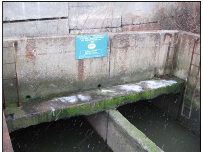
Outfall ID: PR-029 Location: NICHOLAS STREET Latitude: 40° 38' 27" Longitude: 74° 8' 21" Outfall Size: DBL 8'6" X 6' Receiving Water: KILL VAN KULL
