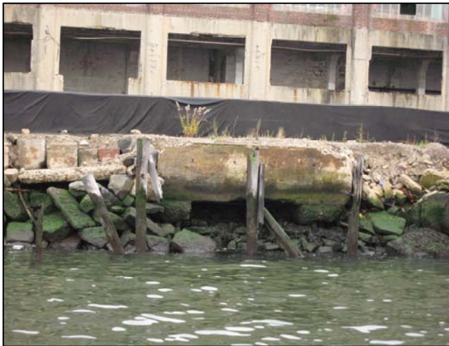
Outfall ID: PR-008 Location: FRANKLIN AVENUE Latitude: 40° 38' 46" Longitude: 74° 5' 35" Outfall Size: 3' X 3' 6" Receiving Water: KILL VAN KULL
