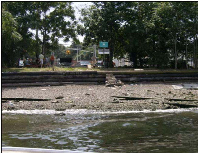
Outfall ID: PR-004 Location: BARD AVENUE Latitude: 40° 38' 44" Longitude: 74° 6' 32" Outfall Size: 18" DIA Receiving Water: KILL VAN KULL
