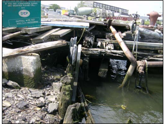
Outfall ID: PR-027 Location: UNION AVENUE Latitude: 40° 38' 17" Longitude: 74° 9' 28" Outfall Size: 12" DIA Receiving Water: NEWARK BAY
