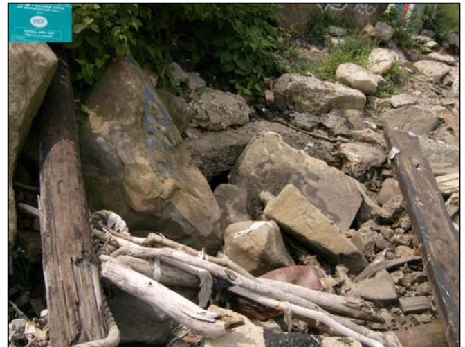
Outfall ID: PR-037 Location: RICHMOND AVENUE Latitude: 40° 38' 28" Longitude: 74° 7' 52" Outfall Size: 5' X 3' Receiving Water: KILL VAN KULL
