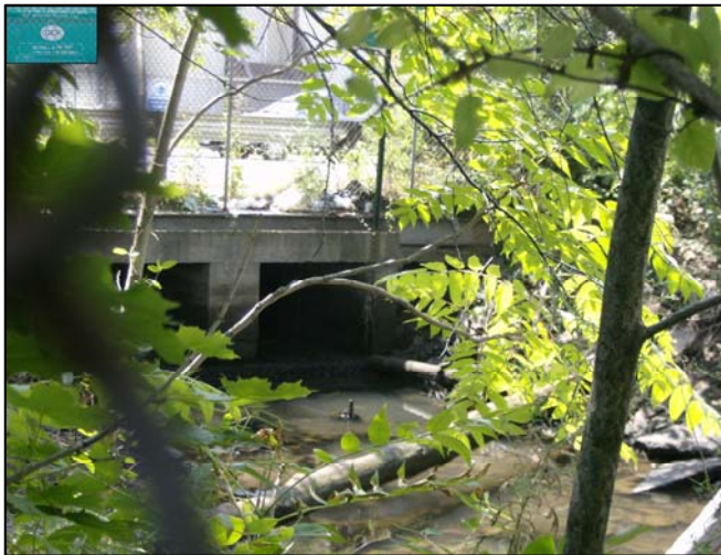
Outfall ID: PR-028 Location: HOUSEMAN AVENUE Latitude: 40° 38' 15" Longitude: 74° 8' 55" Outfall Size: DBL 5' 11-1/2" X 2'9" Receiving Water: NEWARK BAY
