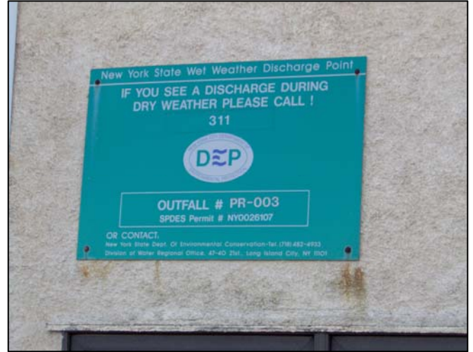
Outfall ID: PR-003 Location: BROADWAY Latitude: 40° 38' 30" Longitude: 74° 7' 6" Outfall Size: 18" DIA Receiving Water: KILL VAN KULL
