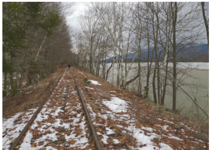
Railroad bed spanning the Northern shore of the Ashokan Reservoir.
