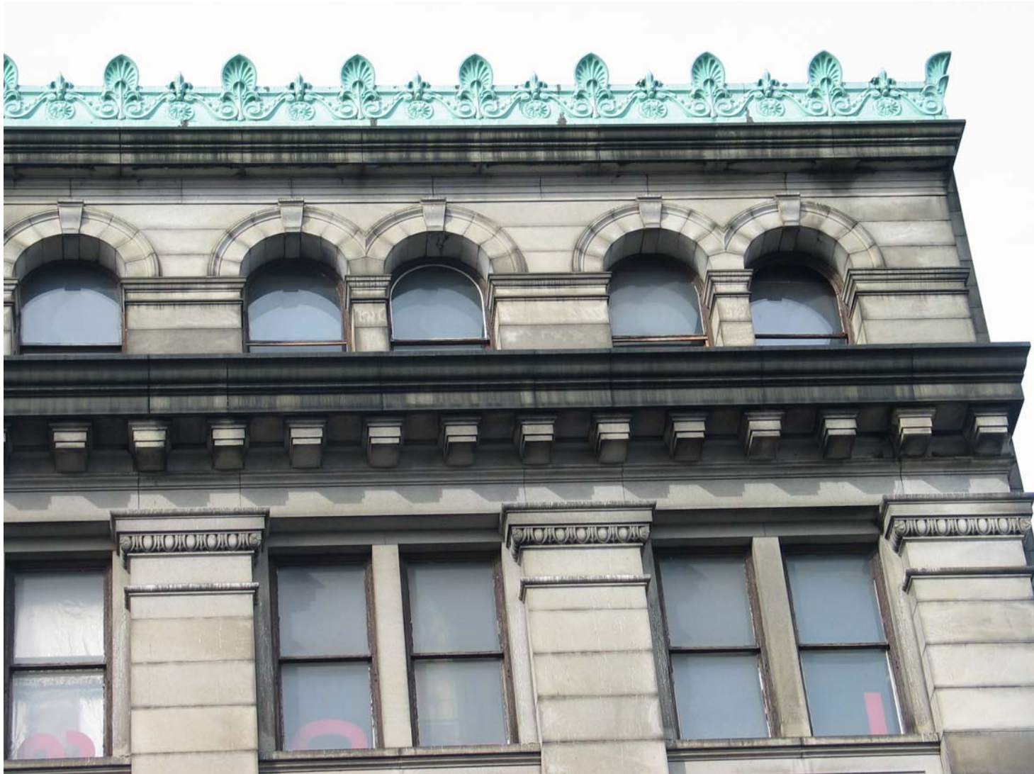
(FORMER) GERMANIA BANK BUILDING , 190 Bowery (aka 1-3 Spring Street), Manhattan. Built 1898-99; Robert Maynicke, architect; Marc Eidlitz and Son, builders. Detail of upper stories and cornice.
