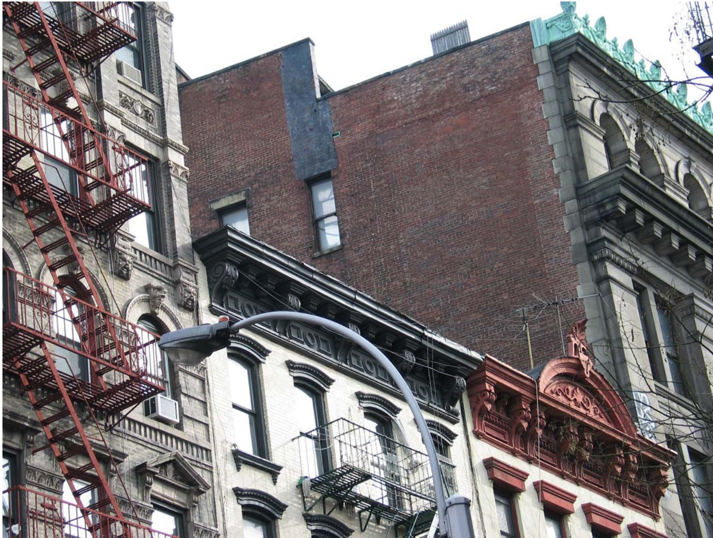
(FORMER) GERMANIA BANK BUILDING , 190 Bowery (aka 1-3 Spring Street), Manhattan. Built 1898-99; Robert Maynicke, architect; Marc Eidlitz and Son, builders. West elevation.
