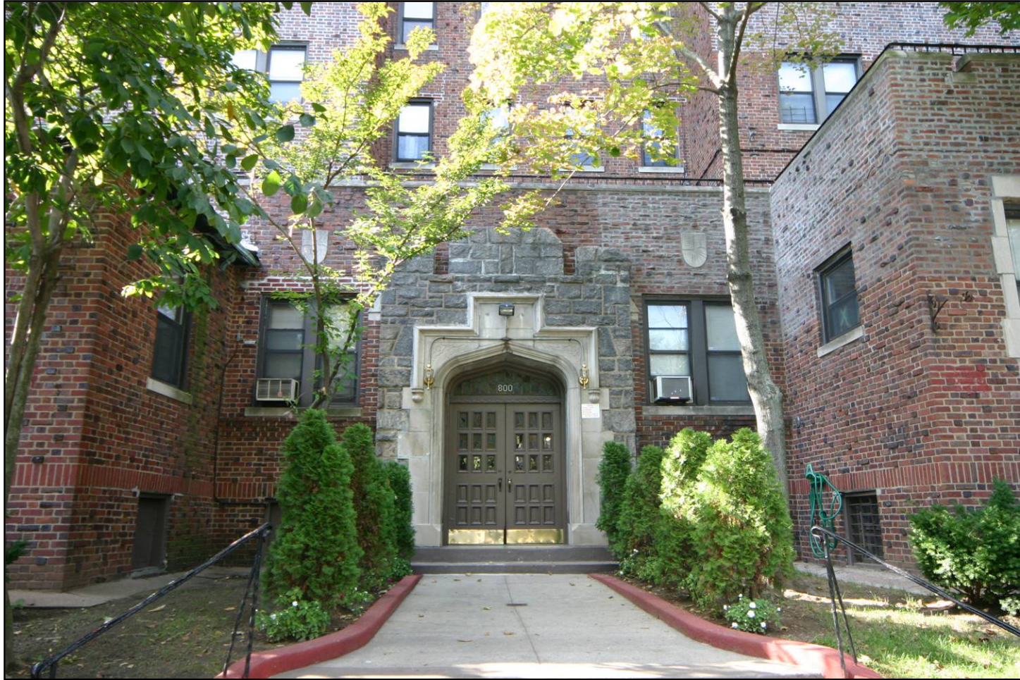
Figure 46 800 East 17 th Street, Entrance Detail James J. Millman, 1936 Photo: Carl Forster
