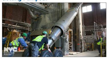
s part of the Water for the Future initiative, last week DEP installed three vertical turbine pumps that will be used to empty the Delaware Aqueduct for the first time since the 1950s. Each of the vertical pumps weighs more than nine tons and stands roughly 23 feet tall. Six centrifugal, submersible pumps will also be installed. The
