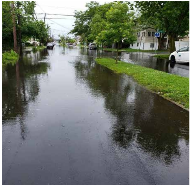
FIGURE 3: EXISTING CONDITIONS AT BEACH-67 STREET, QUEENS
