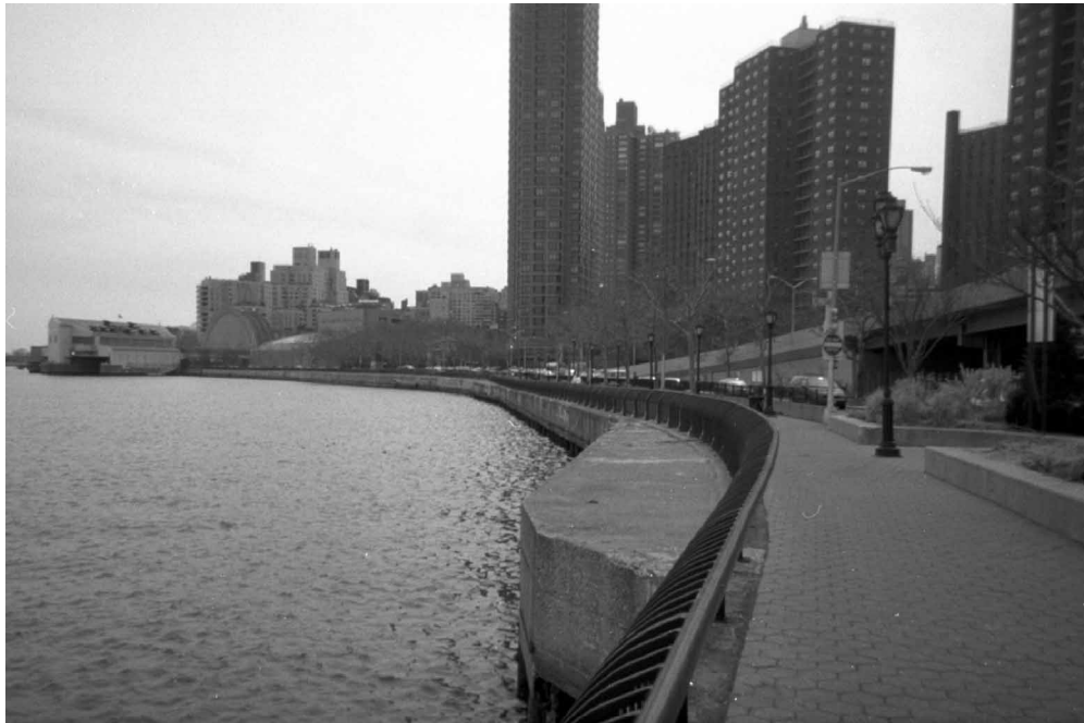
Figure 6.7-6 : View south toward East 91st Street MTS from East River Esplanade at East 96th Street.
