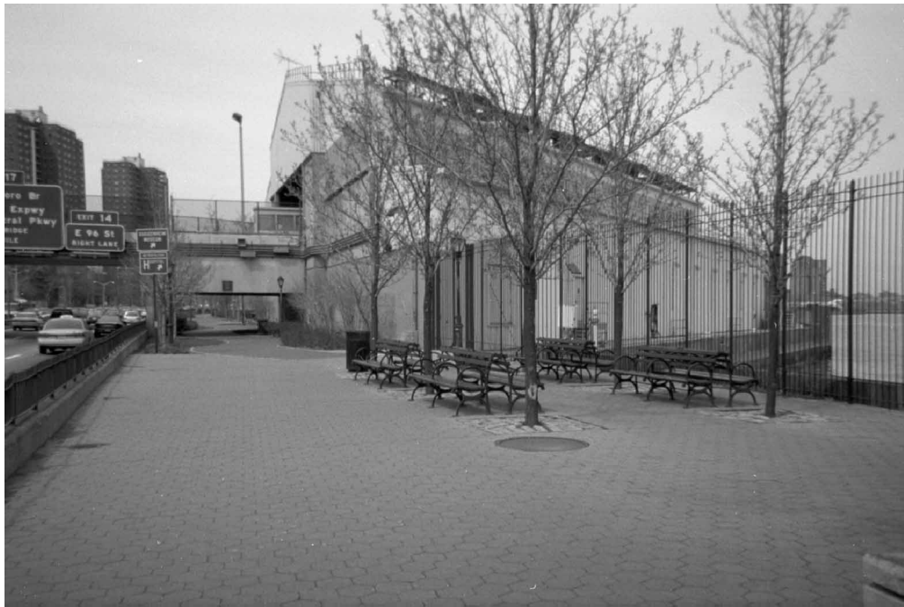
Figure 6.7-1 : View of East 91st Street MTS from adjacent East River Esplanade.
