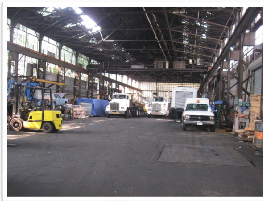
4. Inner view of Building A- Suspect Steel Plates
