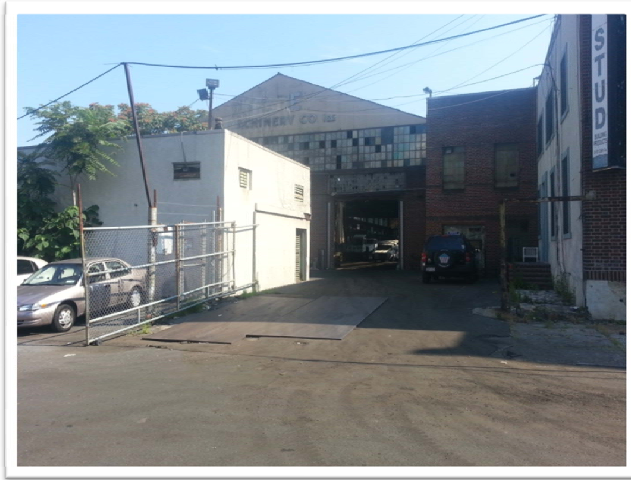
6. Building E- Historical Auto Repair
