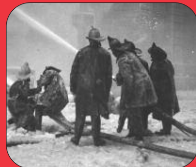
Equitable Building fire, February 1912.
