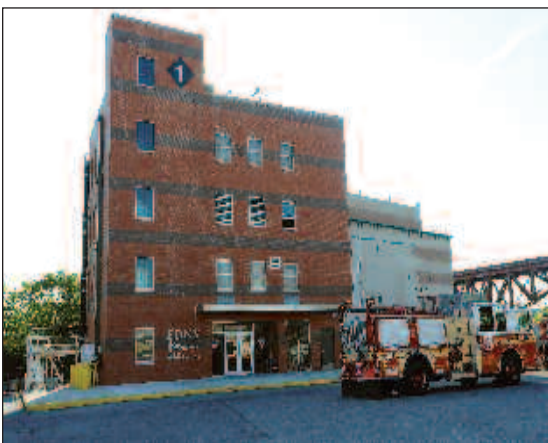
FDNY built several state-of-the-art training facilities at the Randall's Island Training Academy to better prepare Firefighters for any and all emergencies.
