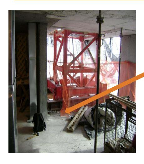
Internal climbing tower cranes require specially designed structural members.
