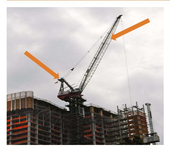
This type of crane consists of "A" frame and boom section mounted on machine platform
