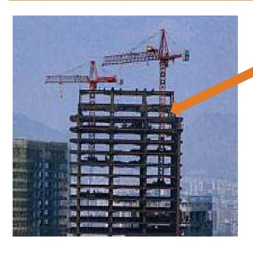
These cranes are installed and attached inside the building through special steel ties.
