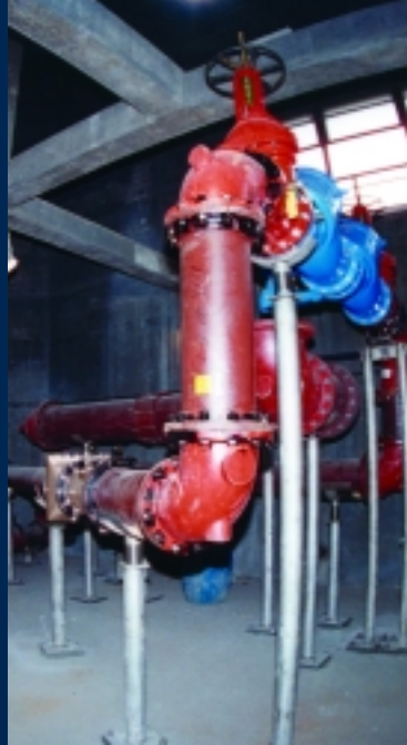
Newtown Creek Sewage Treatment Facility Piping and Meter in Digester
