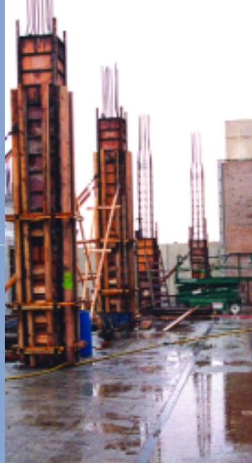
Newtown Creek Sewage Treatment Facility
