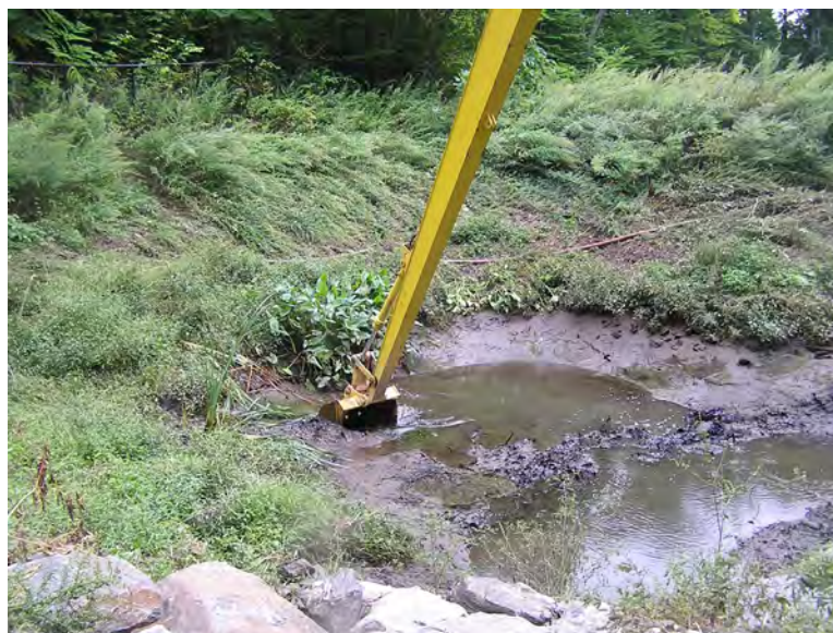
Figure 1.2 Accumulated sediment being removed at BMP 37.
