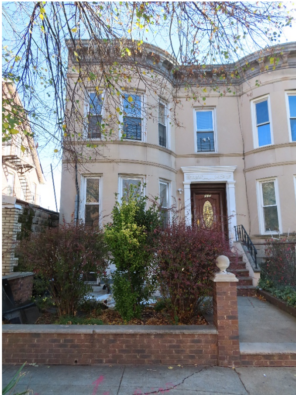
Figure 6: 315 East 25th Street Michael Caratzas, LPC, November 2020
