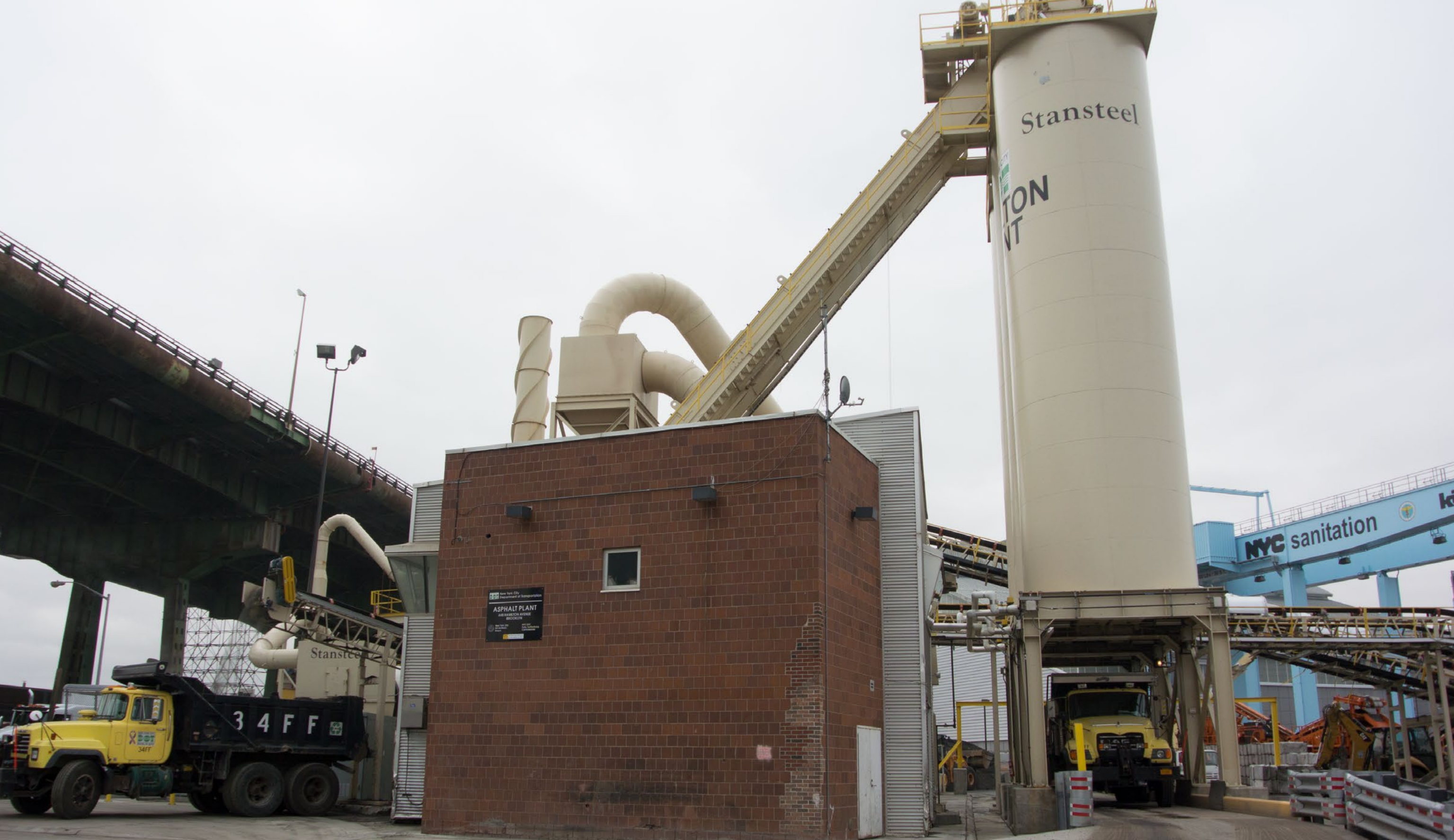
Hamilton Avenue Asphalt Plant Control Tower Renovation
