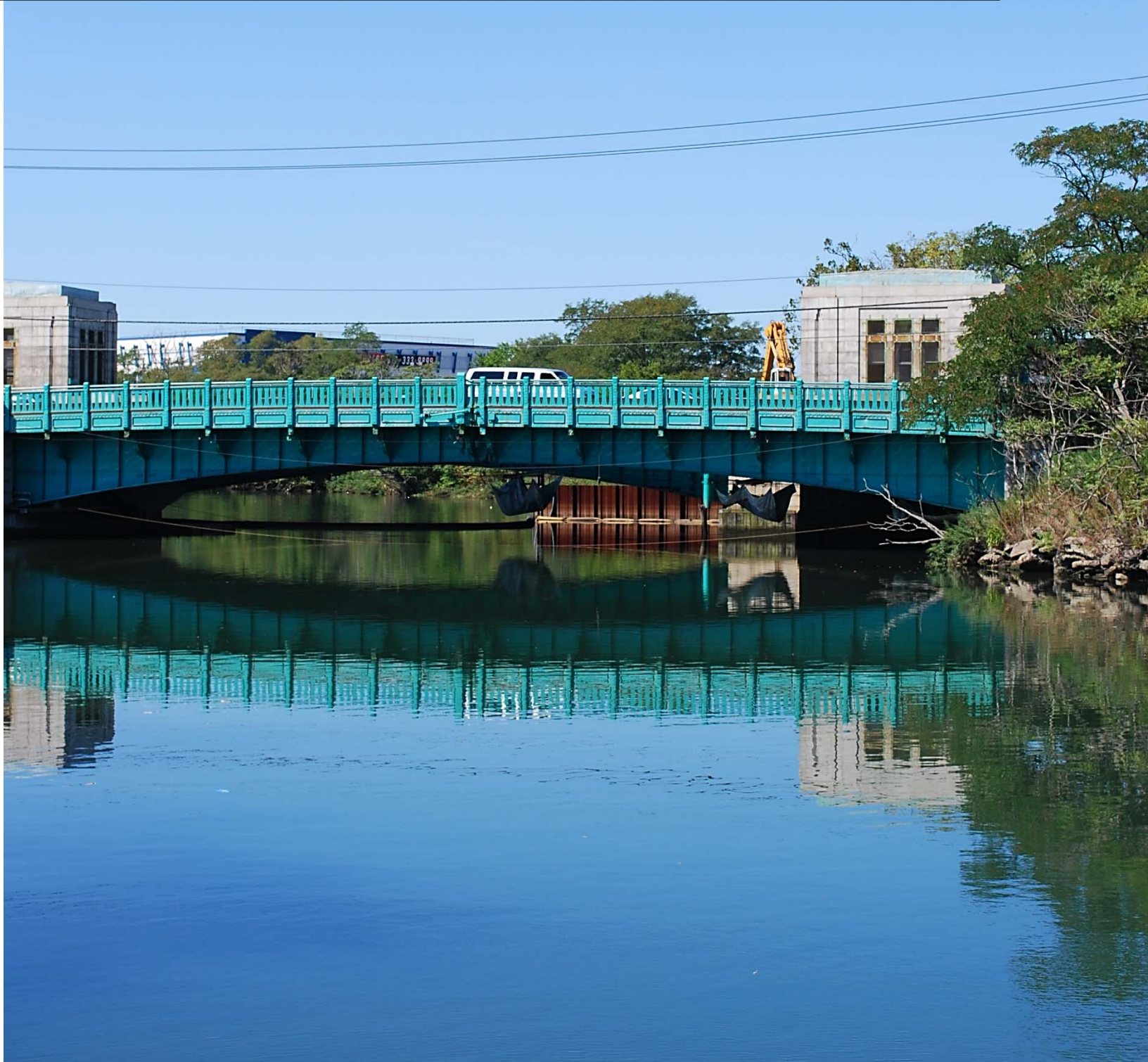
Cropsey Avenue Bridge
