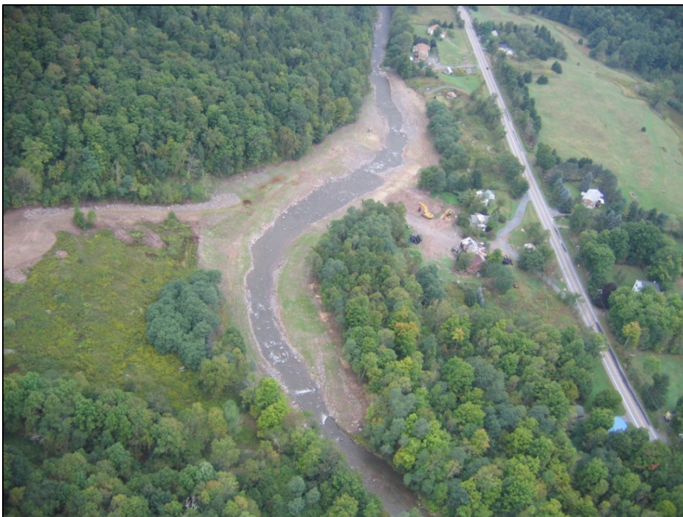
Figure 2-2 Conine Project Post-Restoration, 2009.
