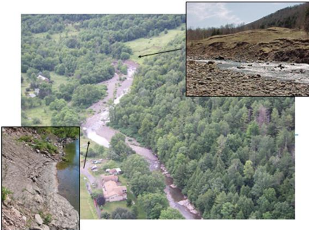
Figure 1-2 The Red Falls restoration project, Phase II proposed area, 2005.
