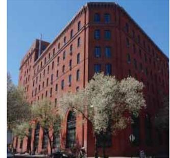
720 Greenwich Street is a 10-story, 157-unit pre-war vaulted brick apartment building. Originally constructed as two warehouses in 1898 and 1902, it was converted into a multifamily building in the 1970s and became a co-op in 1989. Over the years, the building has benefitted from a series of upgrades and ongoing operational improvements that have allowed this one-pipe steam-heated building to achieve superior energy performance.
