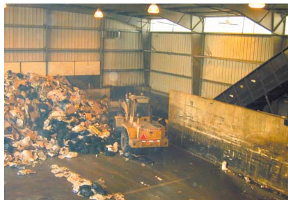
Photo 1-6: Tip floor at the Marlborough facility From the tip floor, a front-end loader moves waste to a conveyor, which feeds to a manual sort line.
