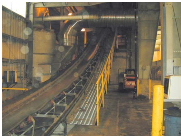
Photo 1-10: Conveyor belt leading to the two-inch, primary trommel screen
