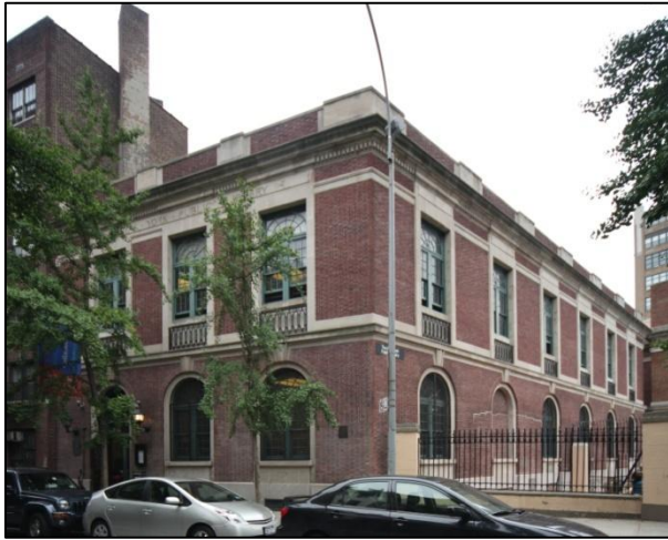
Leroy Street facade
