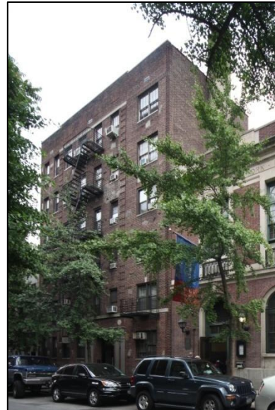
Leroy Street facade
