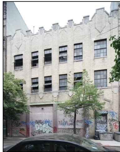
Leroy Street facade
