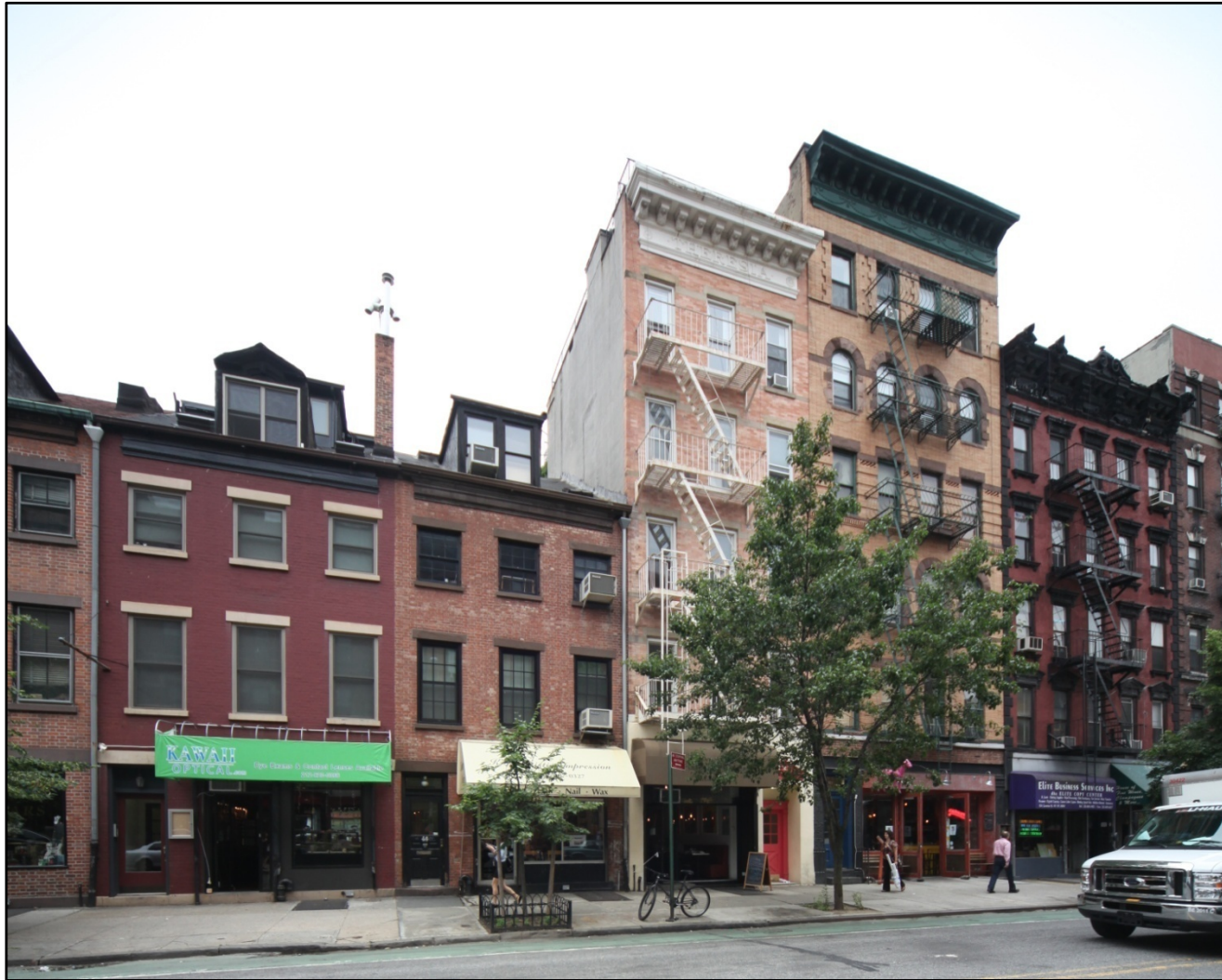
Figure 13: Nos. 44 to 52 Carmine Street, 2010. Photo by: Christopher D. Brazee, 2010.
