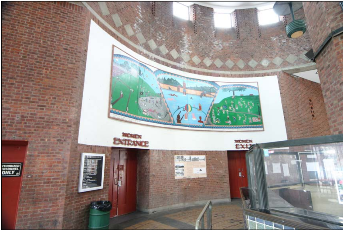
Sunset Play Center Bath House, First Floor Interior Women's locker room entrance and exit doors and wall mural Photo: Carl Forster
