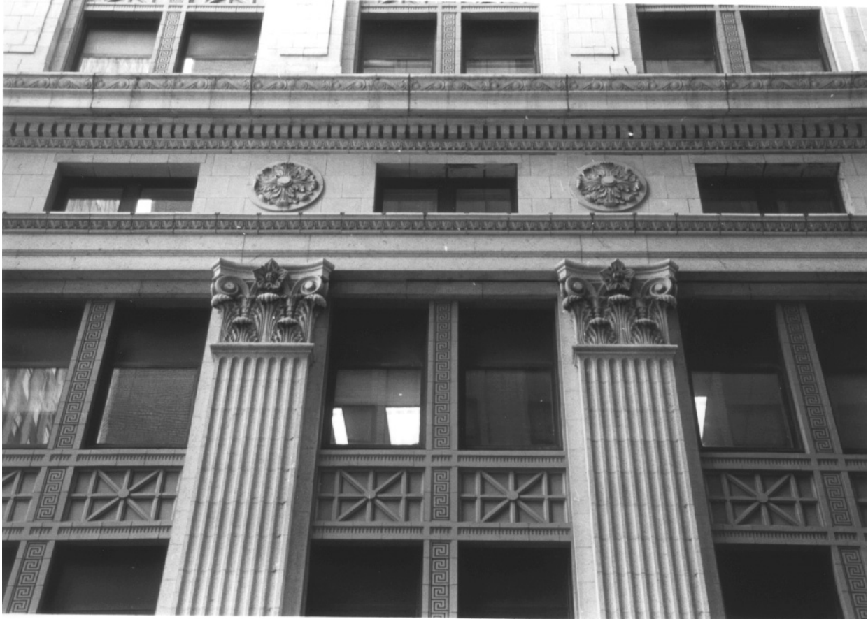
Fig. 6, Detail showing the leaf medallions separating the fourth story window openings Photo: Carl Forster
