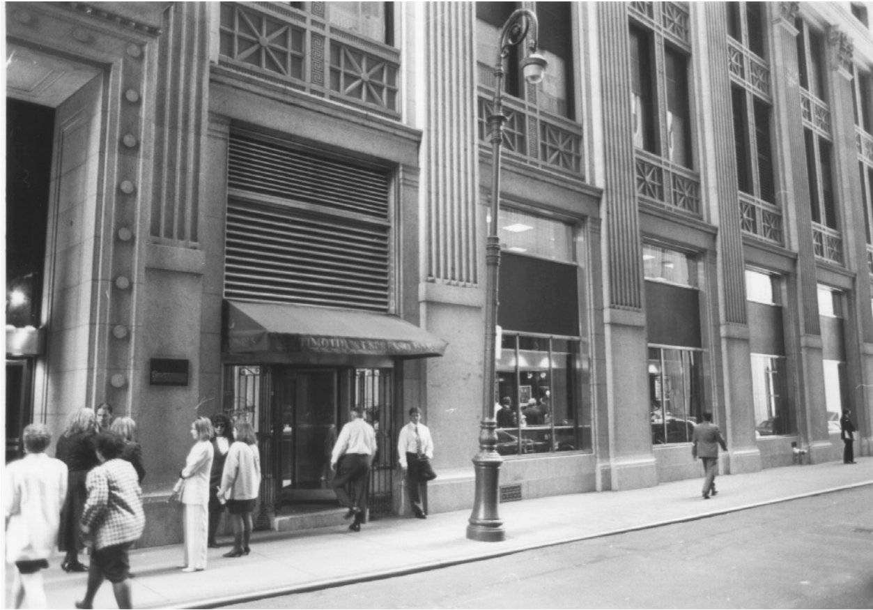
Fig. 12, Ground story commercial entrance and fenestration on Pine Street Photo: Carl Forster
