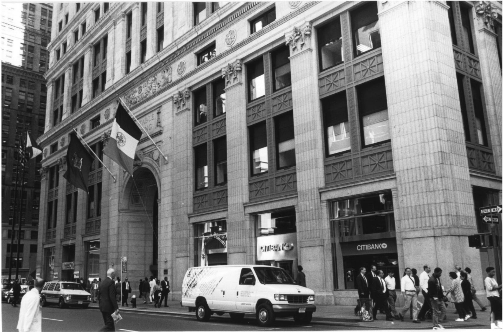
Fig. 4, Base, Broadway façade Photo: Carl Forster
