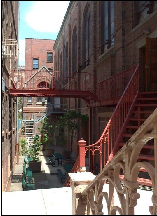
West Facade, West Extension, and Areaway (Photograph: Marianne Hurley, 2016)
