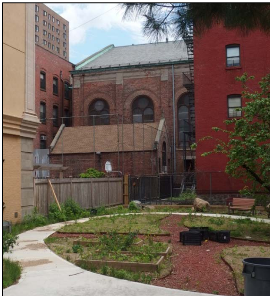
West Facade and West Extension from Park Avenue (Photograph: Marianne Hurley, 2106)
