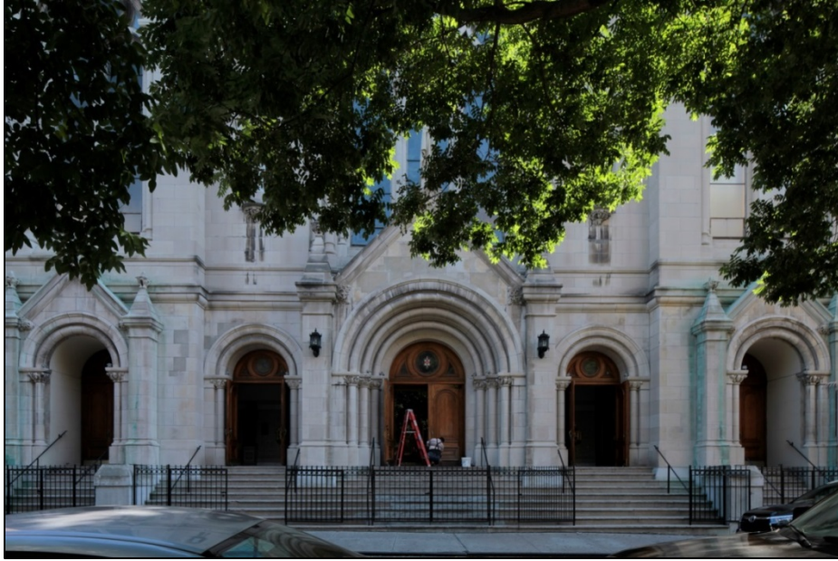
Front Facade 121 East 117 th Street (Photograph: Sarah Moses, 2016)
