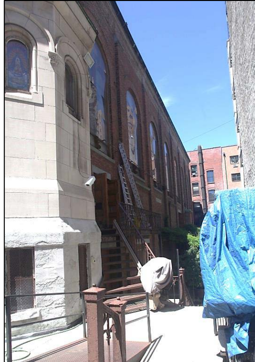
East Facade and Areaway (Photograph: Marianne Hurley, 2016)
