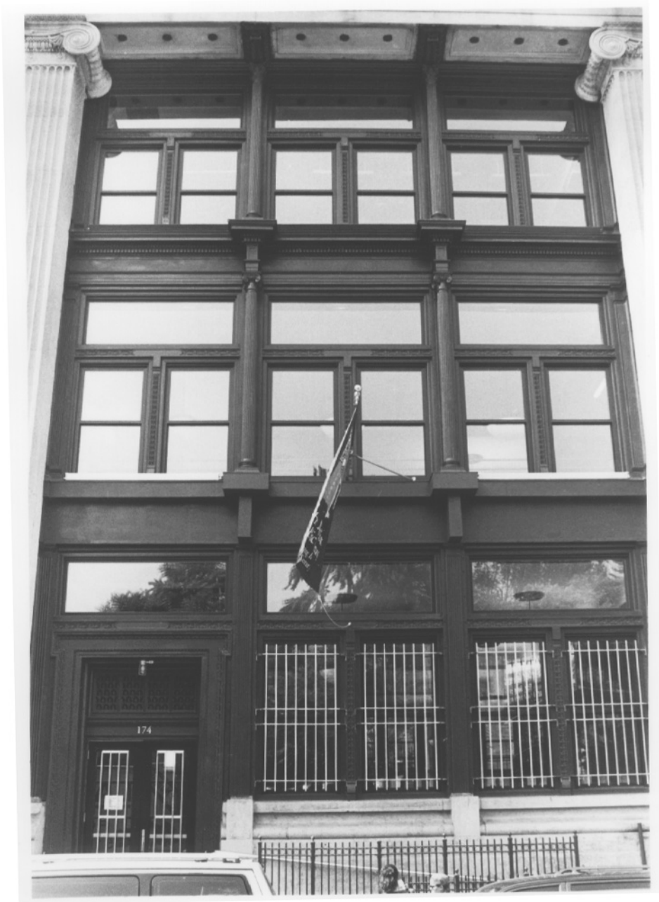
Fig. 5. Detail: Three-story, three bay recessed screen
