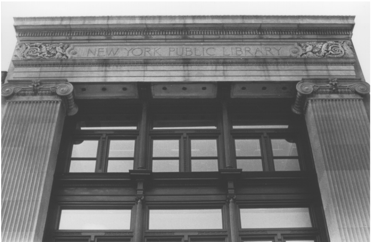
Fig. 3. Detail: Ionic capitals supporting entablature
