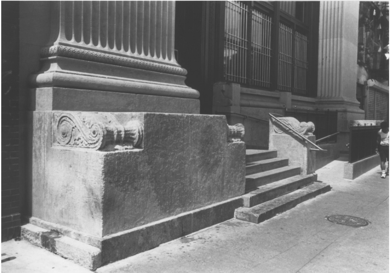
Fig. 2. Detail: Limestone pier on granite base
