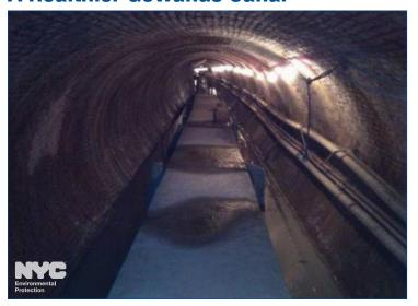
ast week, DEP announced that the Gowanus Canal Flushing Tunnel been reactivated after a full rehabilitation and upgrade that began in 2010. The activation of three submersible turbine pumps is bringing up to 252 million gallons of oxygen-rich water to the head of the Canal each day—or roughly 30 percent more than was possible before
