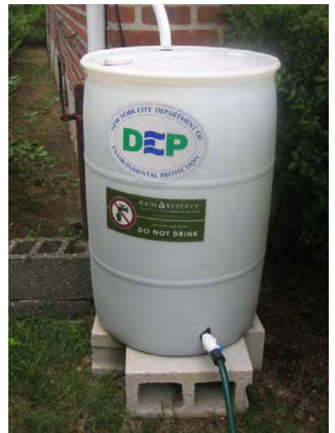
Rain barrel and diverter connected to a homeowner's roof leader
