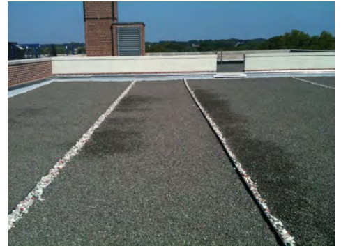
Blue roof portion of rooftop at PS118 constructed with intermediate check dams to
