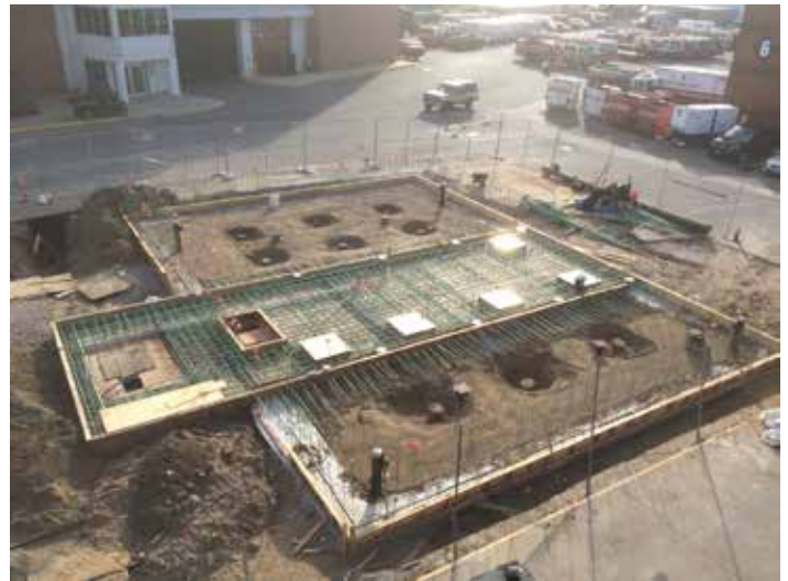
Figure 13: FDNY reuse facility under construction, May 2017
