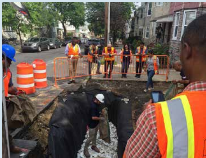
Figure 8: Rain garden under construction with crushed porcelain
