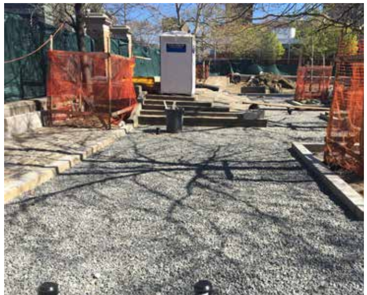
Figure 12: Community Parks Initiative site under construction
