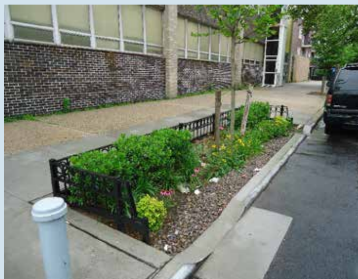
Figure 9: Photo of a completed rain garden
