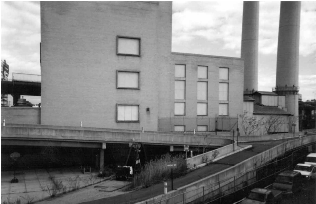
Figure 4.7-2: View of incinerator, facing southeast from the Home Depot parking lot.
