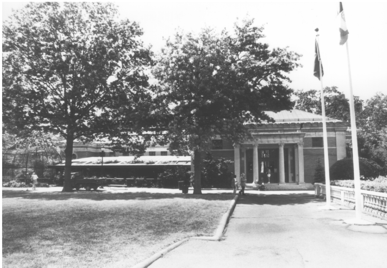
East facade of Large Bird House Photo: Carl Forster
