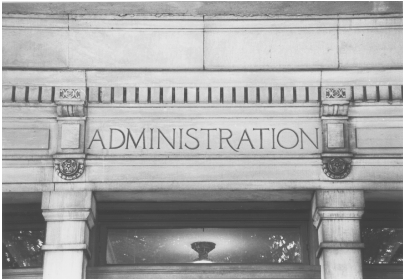
Detail, west facade, Administration Building Photo: Carl Forster
