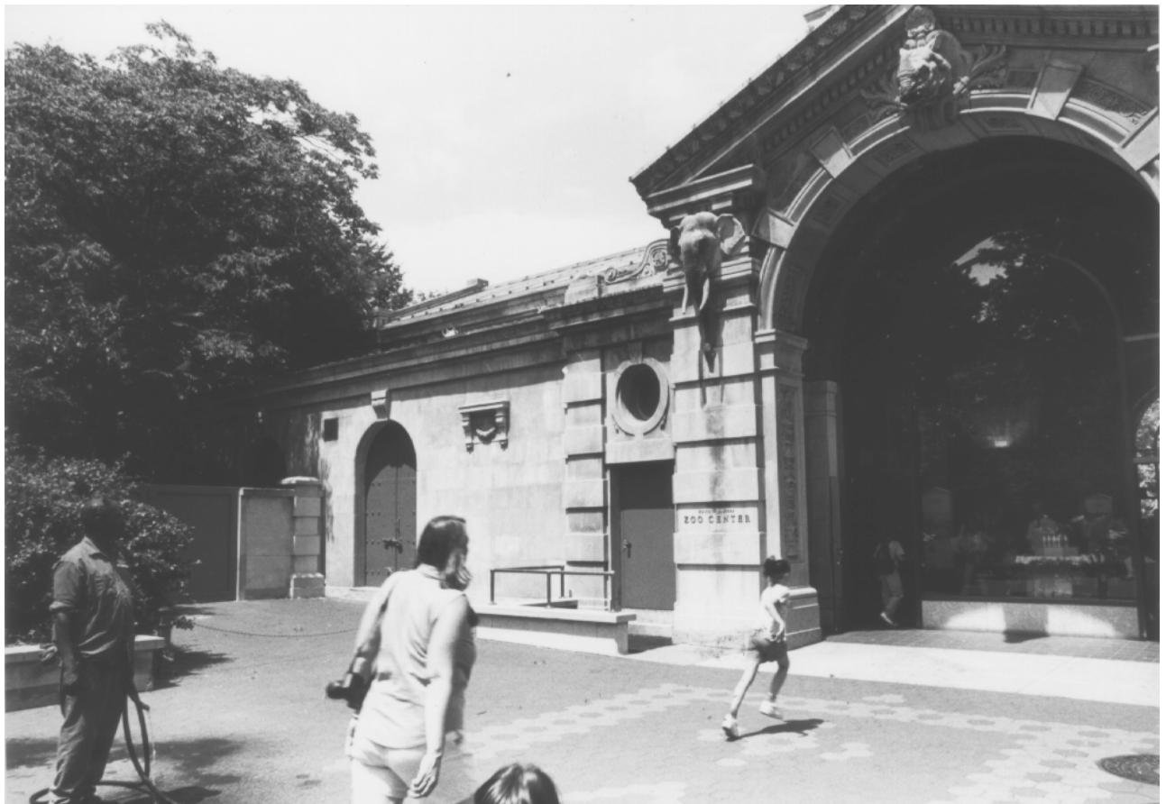
West side of south facade, Elephant House Photo: Carl Forster
