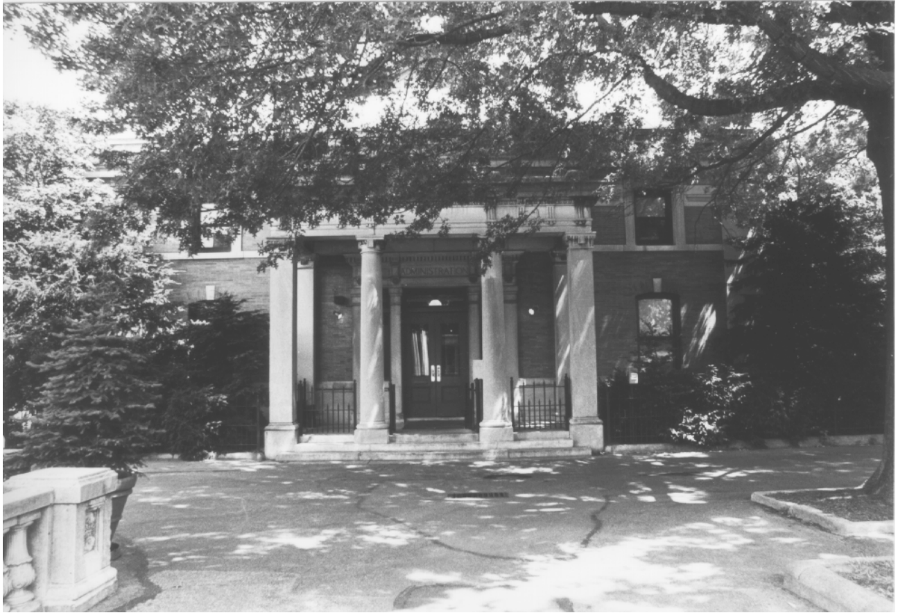
Administration Building, west facade (now Administration East) Photo: Carl Forster
