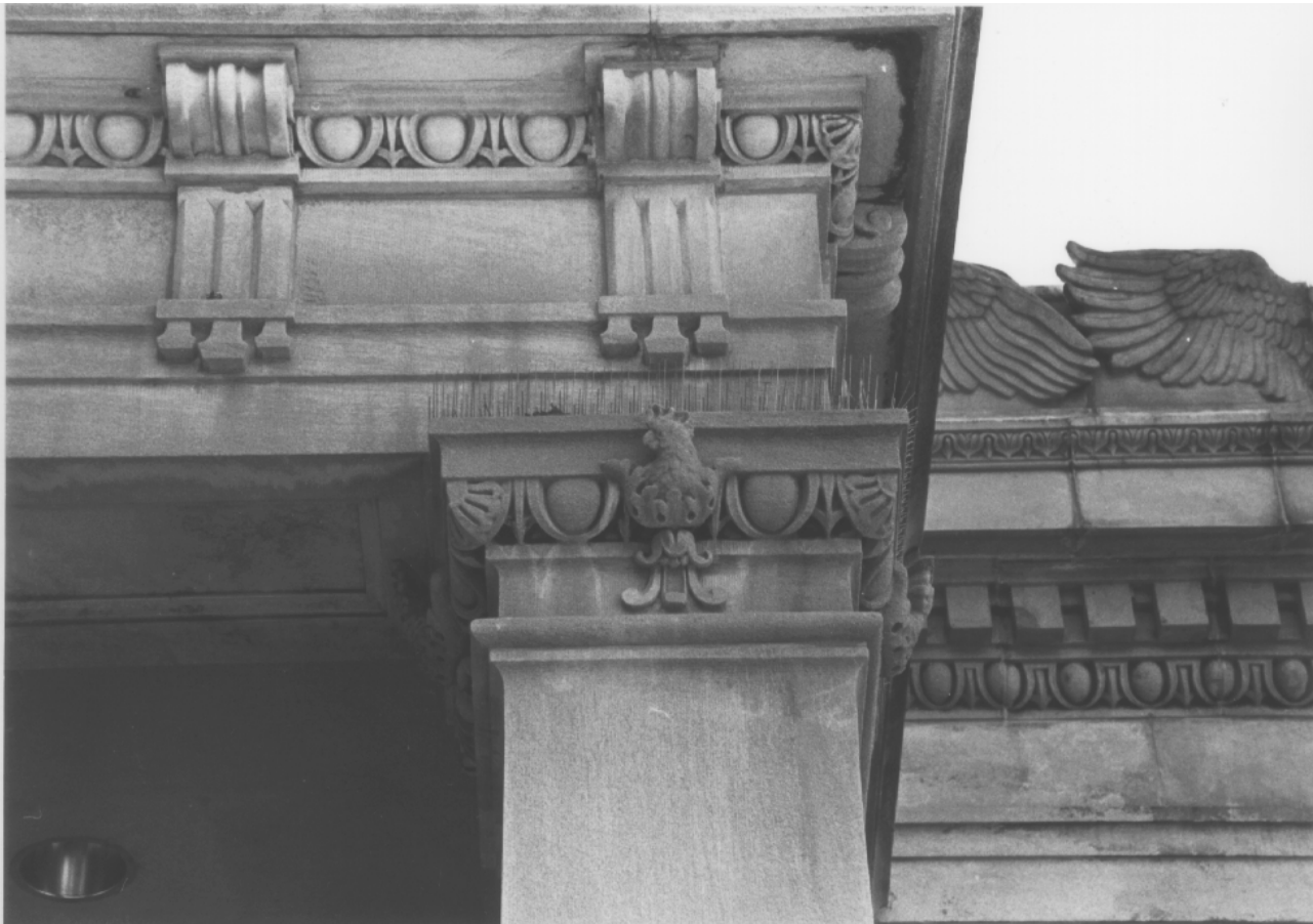
Cockatoo capital and cornice detail, northeast portico of Large Bird House Photo: Carl Forster
