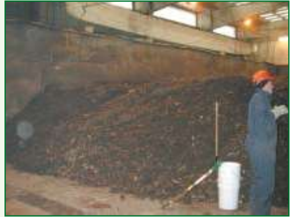
Piles of immature NSS compost begin to “cure” on an aerated floor at the Marlborough facility.
