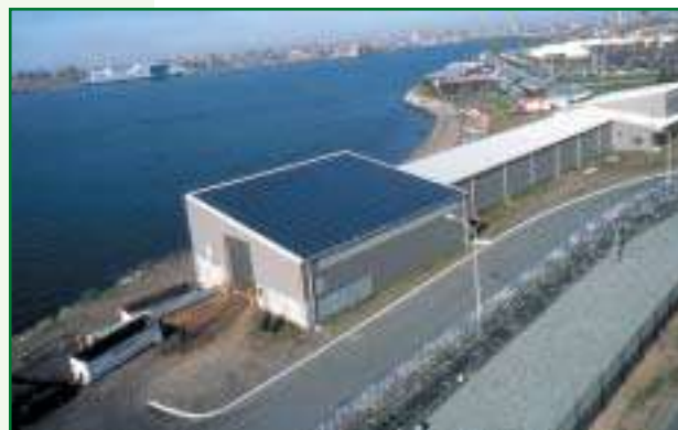
Aerial view of Riker’s Island and the in-vessel, food-waste-composting facility. The facility features the world’s largest installation of a translucent photovoltaic panel roofing system. Installed with funding from the New York Power Authority, the roof panels provide 40 kilowatts of power to the plant.
