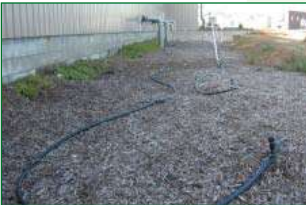
Exhaust air is blown outside the building underground, where it passes up through a biofilter, shown above. Microbes that live in this specially engineered bed of woodchips and compost effectively “scrub” the air of odor-causing compounds. A network of above-ground pipes and sprinklers keeps the biofilter moist.
