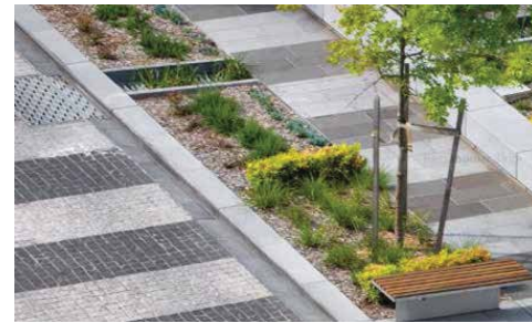
Bio-swale with integrated bench
