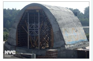
\$21.2 million project to connect the Catskill and Delaware Aqueducts for the first time, a 21-foot tall by 36-foot wide model of the Catskill Aqueduct is currently being built in Orange County. The full scale model will allow contractors to practice drilling large diameter pipe penetrations through the Catskill Aqueduct and ensure that the shutdown
