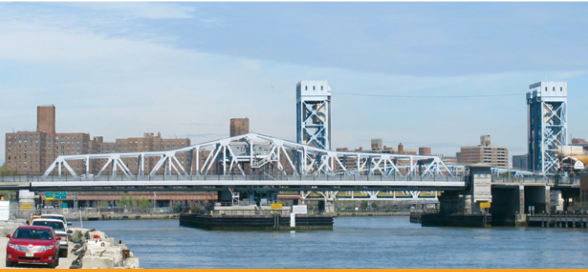
3rd Avenue Bridge
