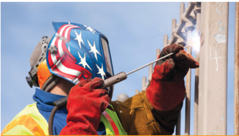
DOT worker fixing Brooklyn Bridge
