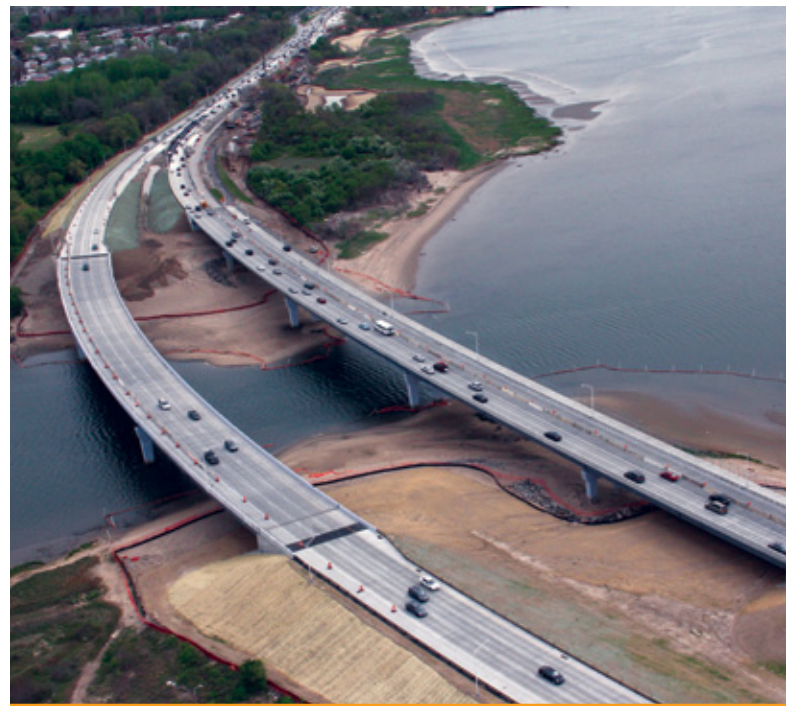
New Paerdegat Basin Bridge in Canarsie.
