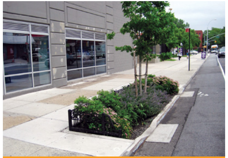
Bioswales use planted areas to reduce drainage
