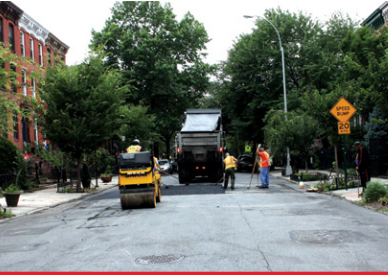
Speed bump installation
