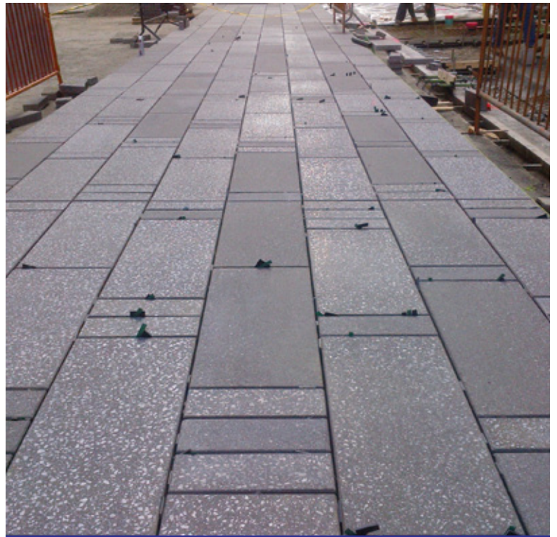
Pavers being installed as part of Times Square reconstruction project
